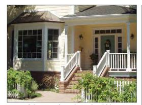
Original doors and windows should be retained and repaired
