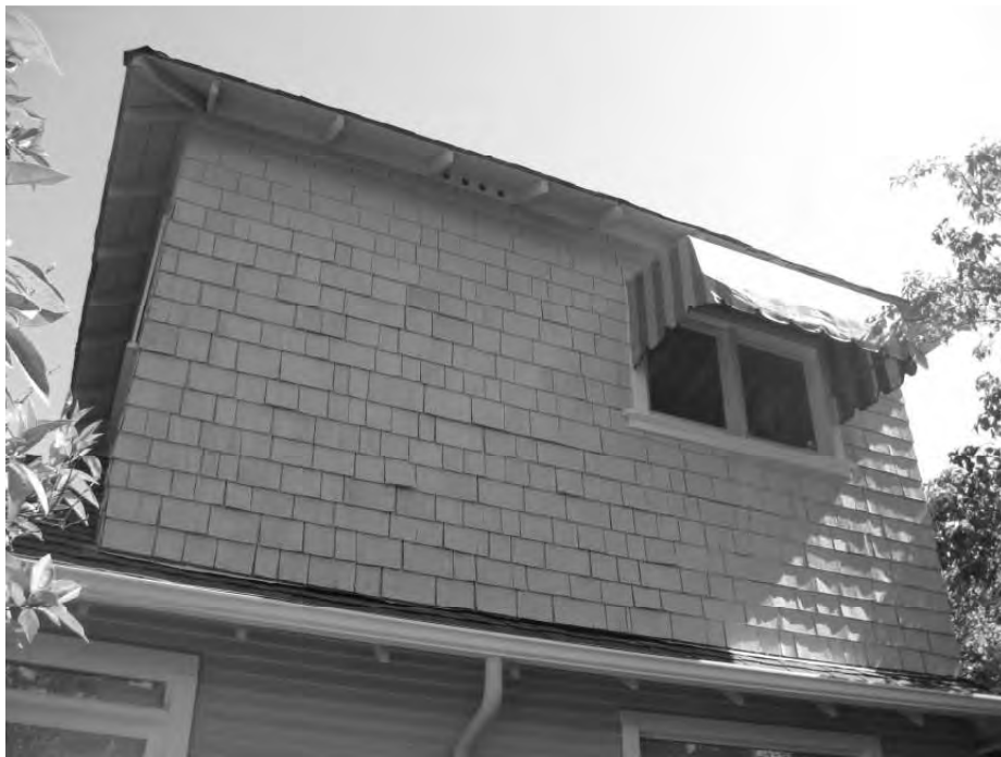
Photo 10: View of the 2 nd story, rear façade.
