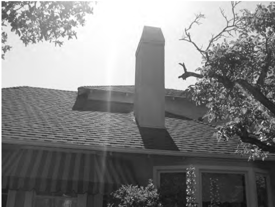
Photo 7: Detail of the (non-original) chimney.
