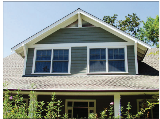
Heavy profile fireproof composition shingles may be used as a replacement for wood single and wood shake roofs
