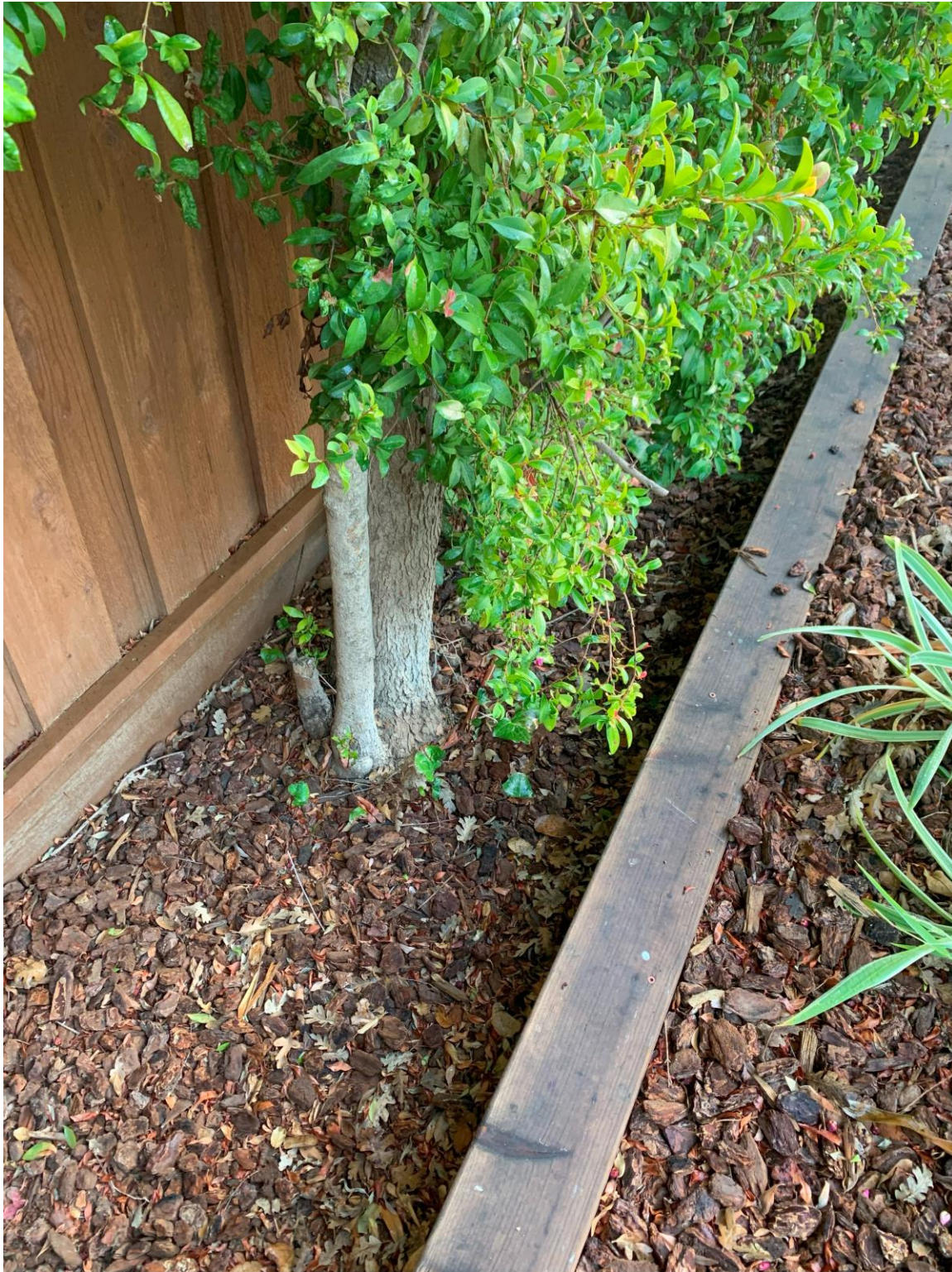
Figure 1: This photo shows the immediate loss of 1-1.25 feet of fence height within 2' of the rear fence as the remainder of the yard is raised at this point and then continues to slope up towards the house.
