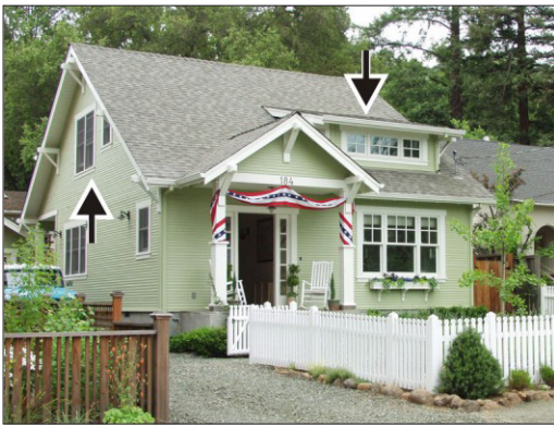
Addition incorporated into the roof successfully adds space while respecting the integrity of the existing house and the scale of the neighborhood
