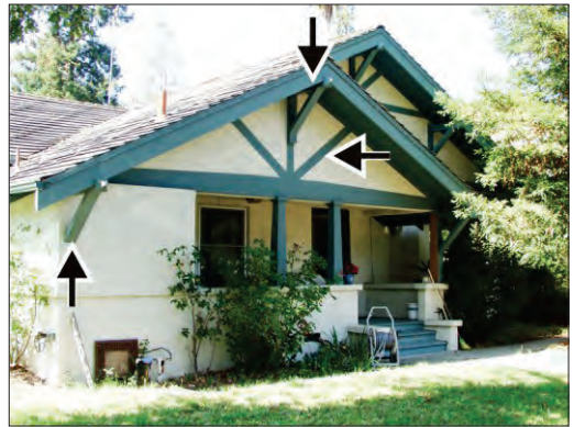
Restore gable and eave details, but don't add features that were not original to the house
