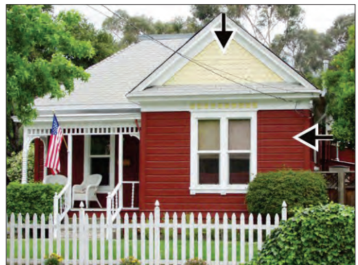
Maintain the siding scale and patterns of the original structure
