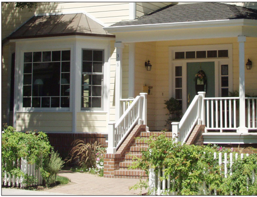
Original doors and windows should be retained and repaired
