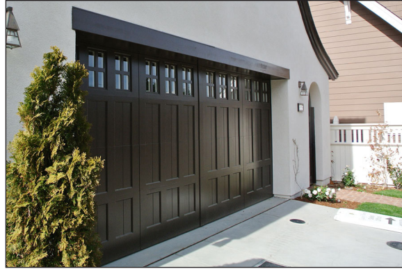
Recessed garage doors
