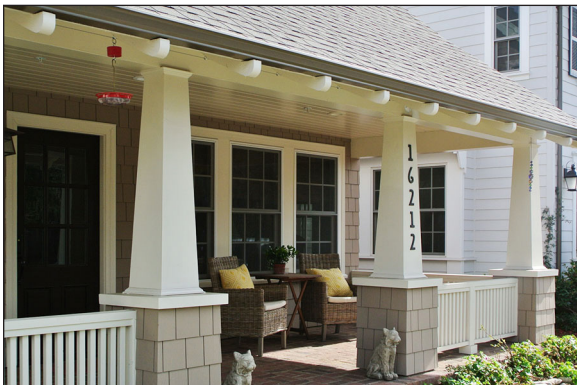
Porch beams and columns
