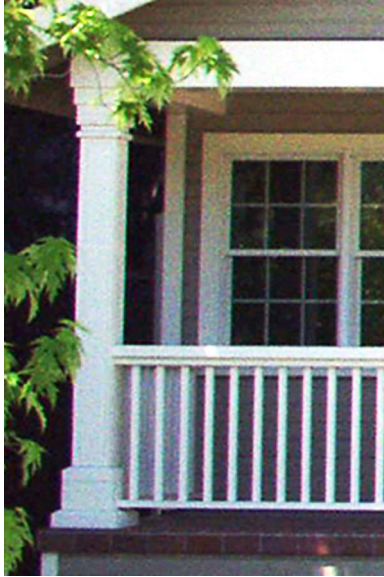
Wood columns and beam
