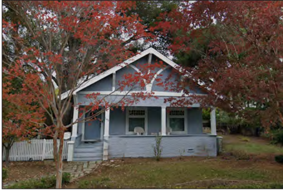
The Site: Street Frontage
