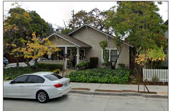
Nearby house Across Tait Avenue
