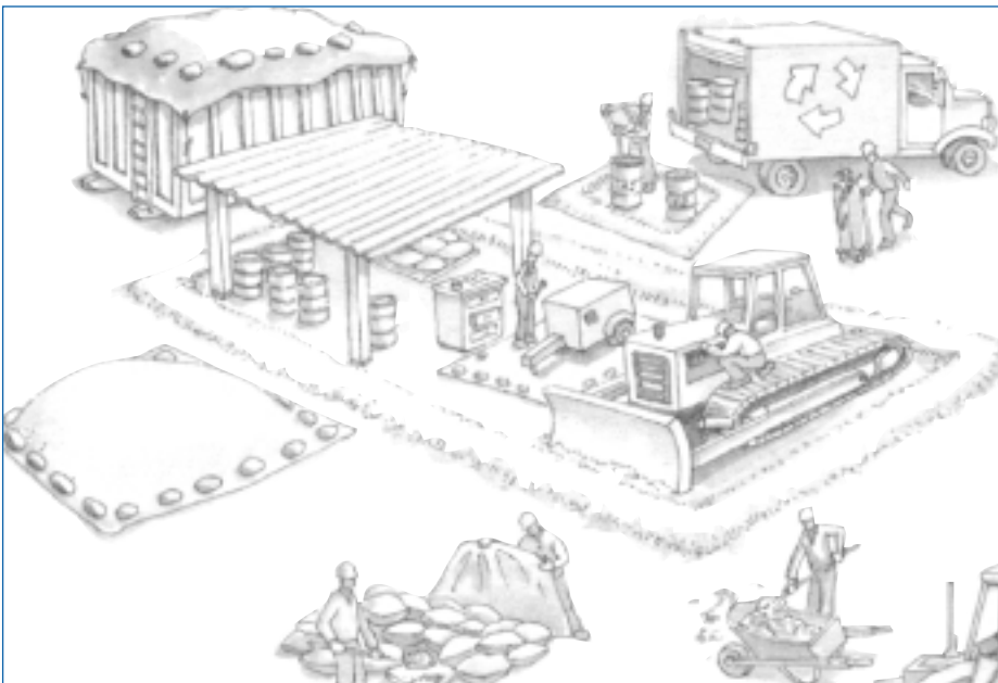
Store building materials under cover. Make sure dumpsters are properly covered to keep out rain.
