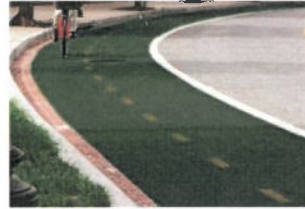
TONED AC PAVING FOR THE TRAIL ALONG EVA
