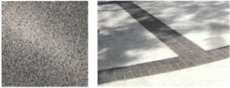
VEHICULAR PAVER BAND – 8"X8"X3" THICKNESS GRANITE PAVERS AT ARRIVAL COURT MFR: COLD SPRING GRANITE COLOR: ACADEM BLACK FINISH: THERMAL
