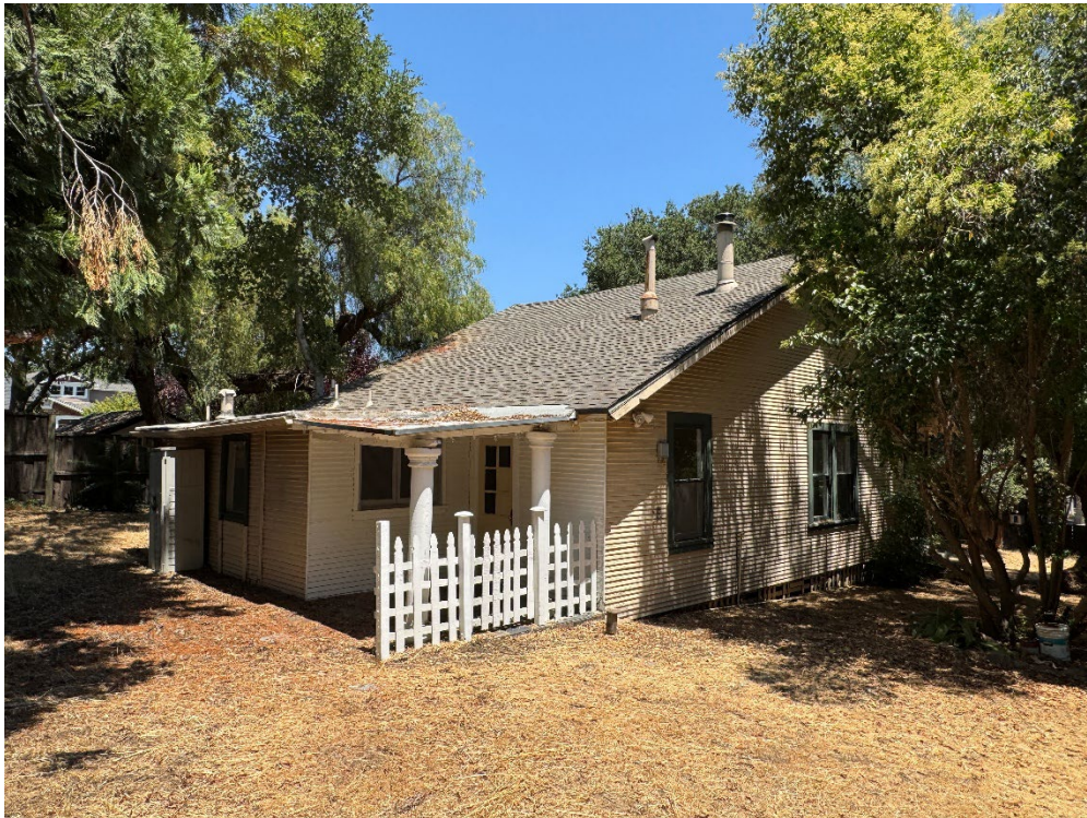
651 N. Santa Cruz Ave. View: West facade Note extensive alterations extending the roof to cover additions, and with Neo-classic architectural columns from other eras that remove the Craftsman style character.
