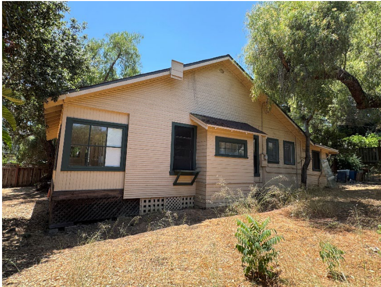
651 N. Santa Cruz Ave. View: North facade with shed pop out. Note the additions on the left and right sides of the building.
