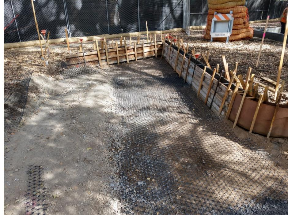
Above right: Close-up image of a WALCA project at Stanford where TriAx TX160 triaxial geogrid was used as a geogrid underlayment over the soil surface, to allow the construction to proceed as a “no dig” system where no subbase prep was performed at all. The grid was laid over the existing soil surface, and baserock and asphalt laid directly over that baserock after the baserock was compacted to a 90% or 95% rate.
