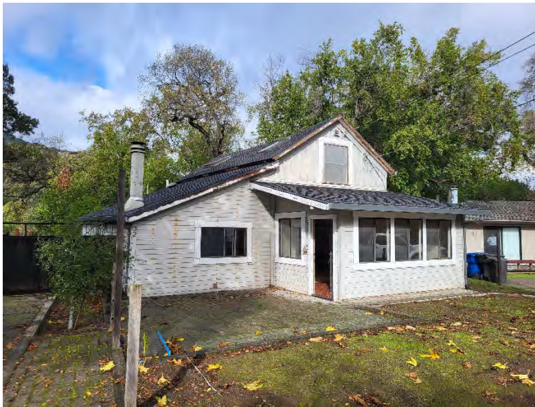
Figure 2. Overview of 32 Euclid Avenue. (view northeast; January 10, 2024)
