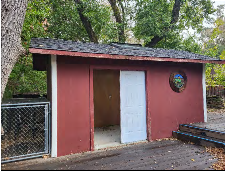
Figure 8. 32 Euclid Avenue Shed (view north/northwest; January 10, 2023).
