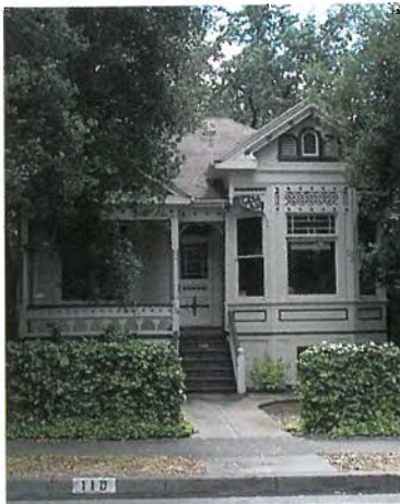
THE MACABEE HOUSE is Eastlake-style, identified by the turned wood columns on the porch and the turned pendants.
