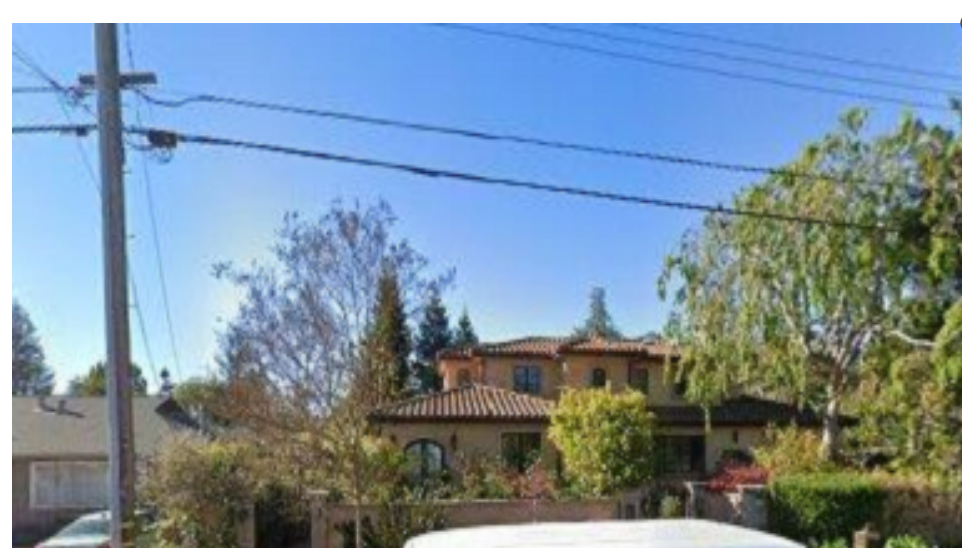
394 Cuesta Dr, Los Altos, HOUSE STYLE: SPANISH NUMBER OF STORIES: 2 EXT. MATERIALS: STUCCO ROOF STYLE: HIP/GABLE ROOF MATERIALS: TILE
