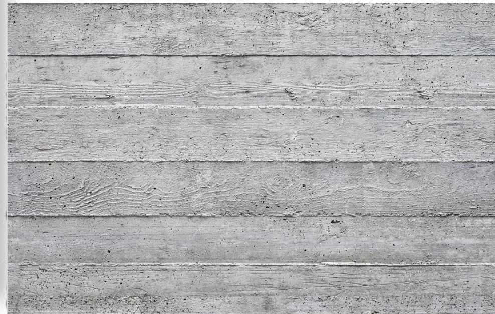
BOARD-FORM CONCRETE LANDSCAPE WALLS
