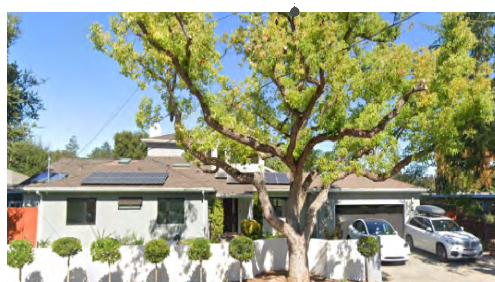
483 Cuesta Dr, Los Altos, HOUSE STYLE: TRANSITIONAL NUMBER OF STORIES: 2 EXT. MATERIALS: STUCCO ROOF STYLE: GABLE/HIP ROOF MATERIALS: COMP SHINGLE
