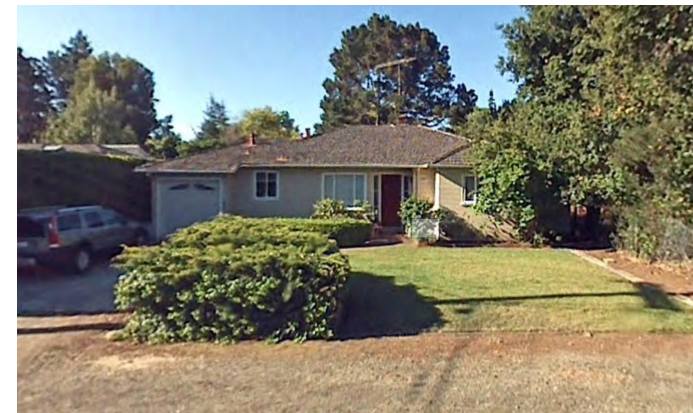
474 SAN LUIS AVENUE HOUSE STYLE: TRADITIONAL NUMBER OF STORIES: 1 EXT. MATERIALS: WOOD ROOF STYLE: HIP ROOF MATERIALS: SHAKE
