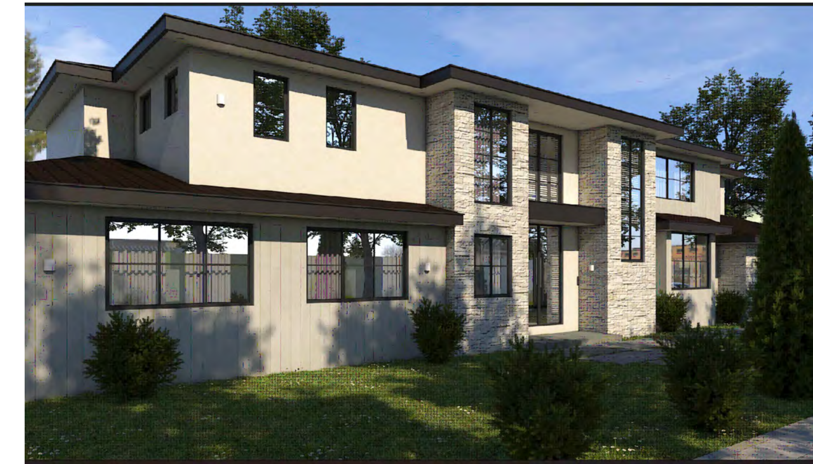
3 FRONT SOUTH WEST FACADE
