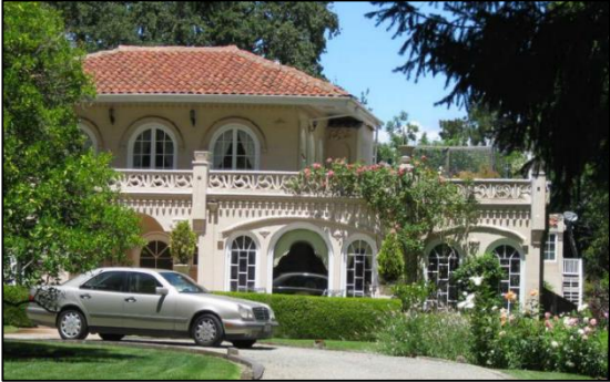
Figure 1: Existing Historic House
