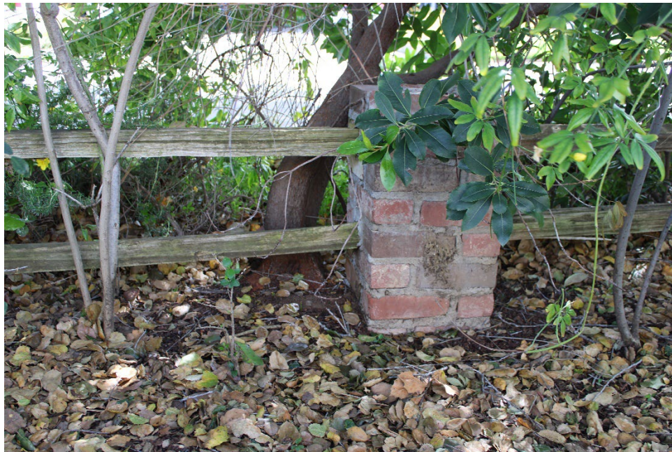
Figure 14. Fence with brick posts and wood rails along southern perimeter of the property.
