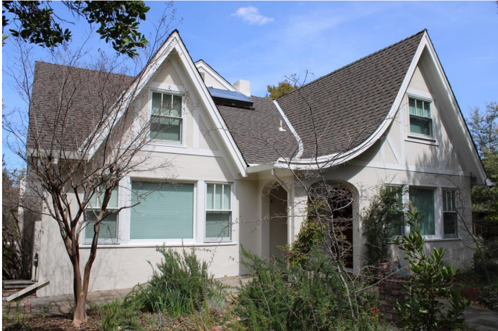
Figure 30. South elevation, facing northeast.
