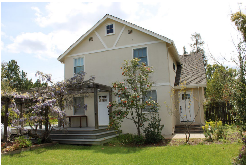
Figure 8. North elevation, facing south.
