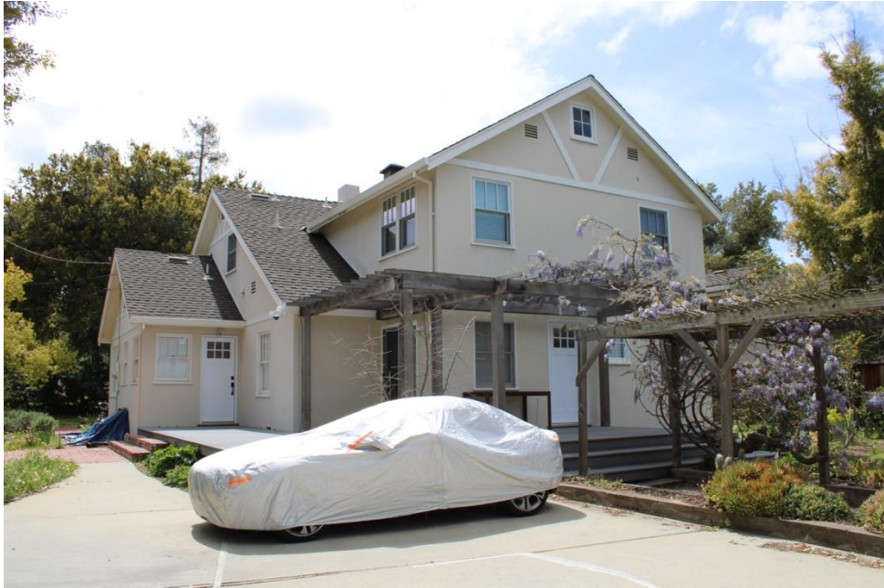
Figure 35. North elevation, facing south.
