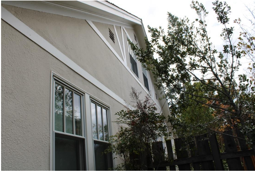
Figure 37. West elevation, facing southeast.
