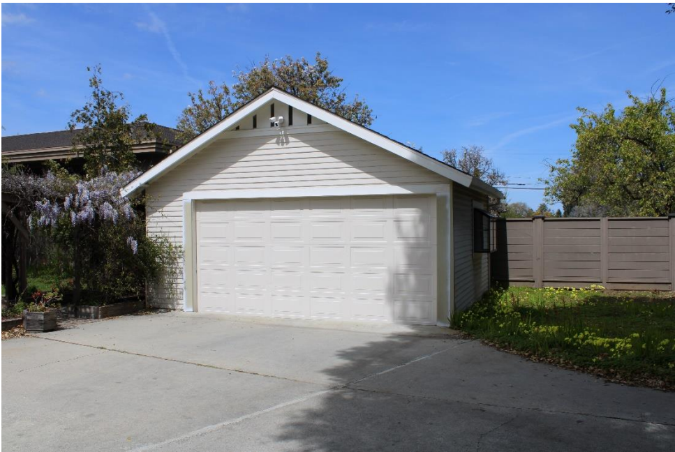
Figure 39. South elevation of detached garage, facing north.
