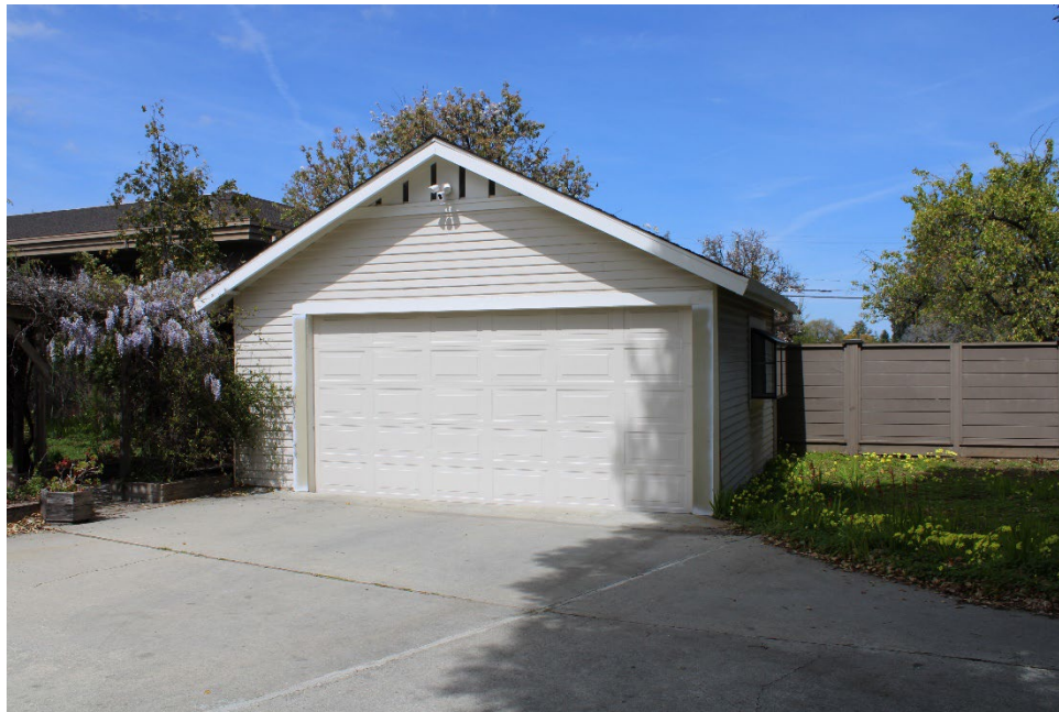
Figure 11. South elevation of detached garage, facing north.
