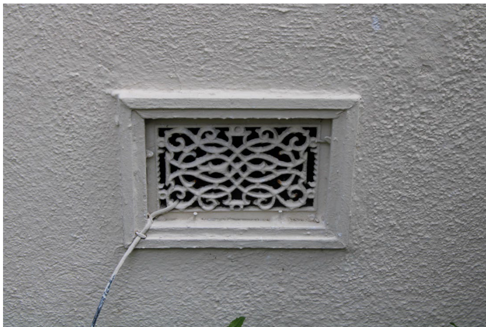
Figure 10. A cast-iron vent cover, along the foundation wall.
