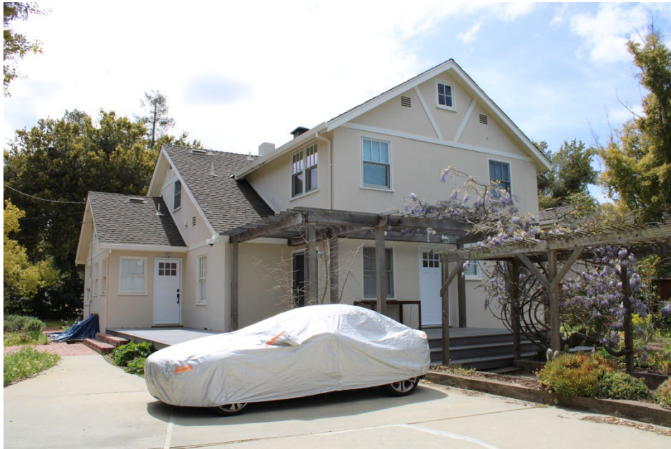
Figure 7. North elevation, facing south.
