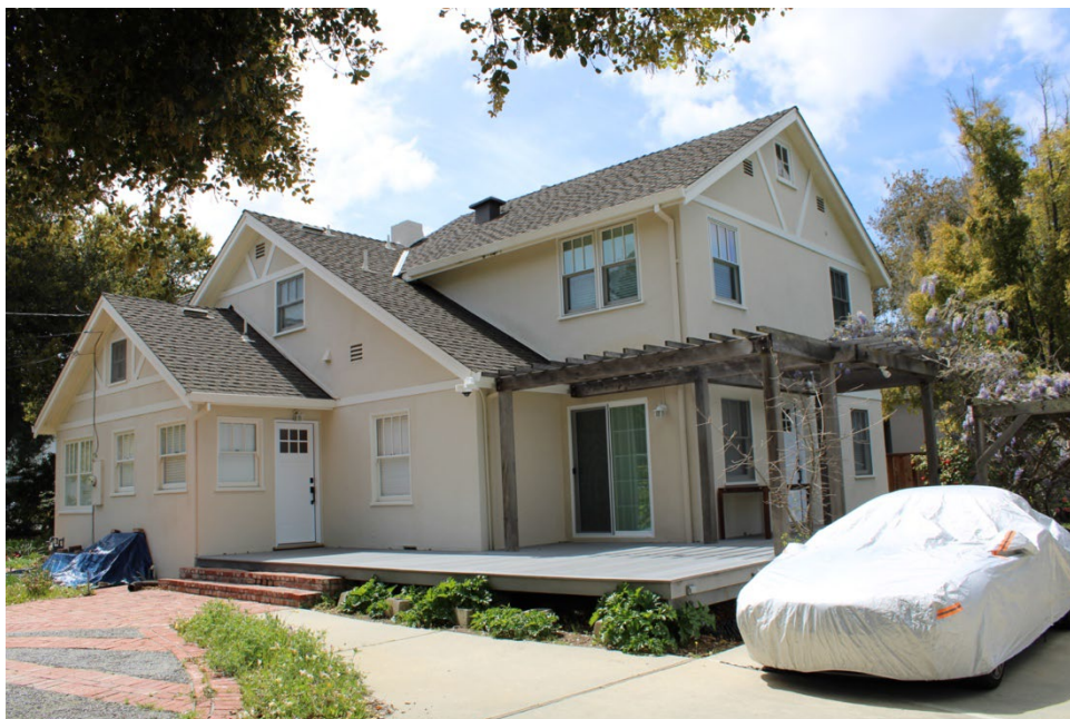
Figure 6. East elevation, facing southwest.
