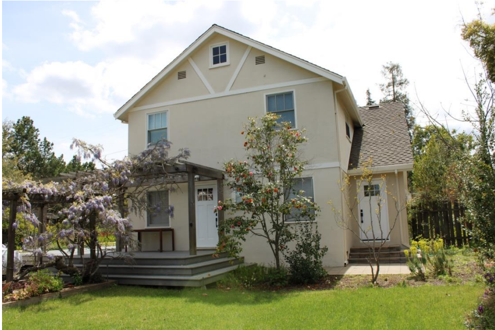
Figure 36. North elevation, facing south.
