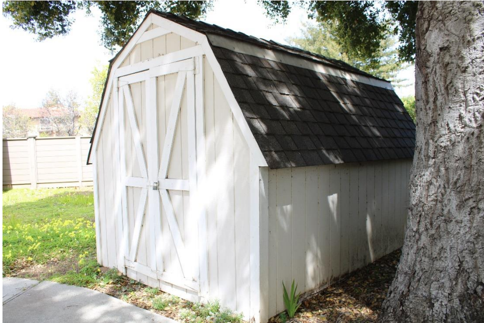
Figure 41. Photograph showing the double-entry doors along the southwest elevation (primary façade) of the ca. 1980 storage shed, facing north.
