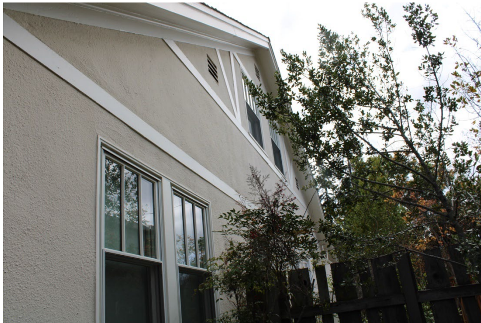
Figure 9. West elevation, facing southeast.
