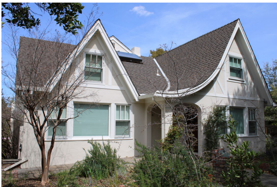
Figure 2. South elevation, facing northeast.
