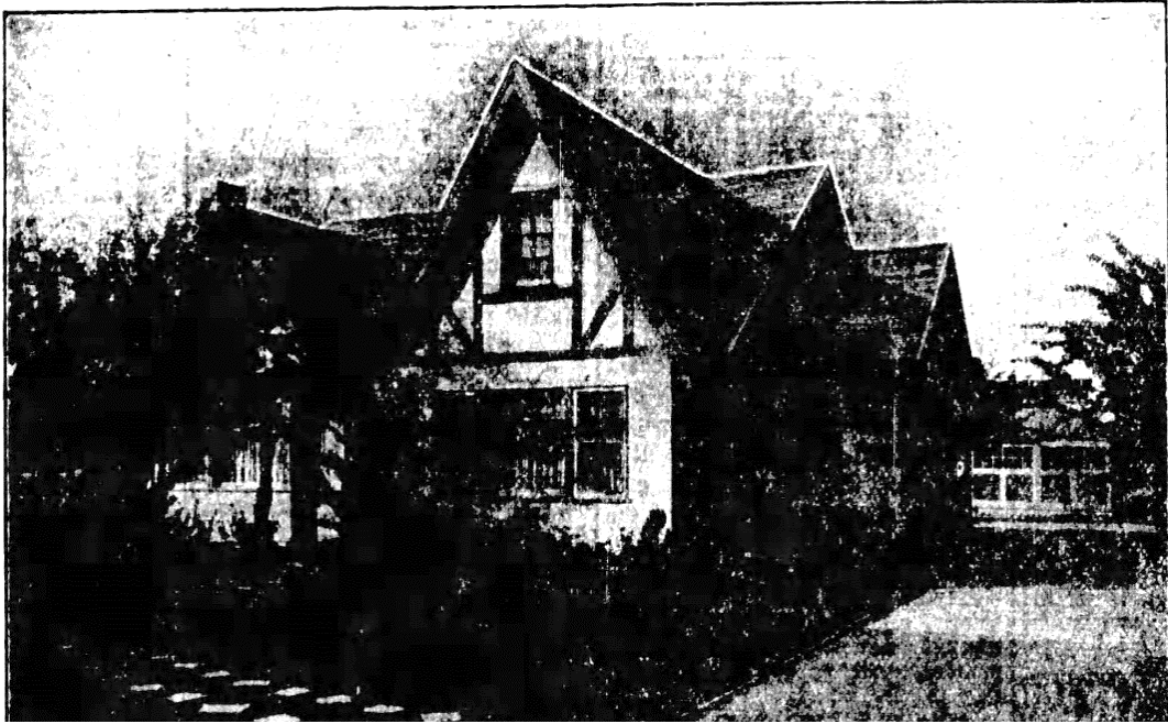
Figure 17. A 1927 newspaper photograph of the 1926 house with the rectangular detached garage (no longer extant) at the rear of the property (courtesy of Newspapers.com, The Daily Palo Alto times, December 3, 1927).
