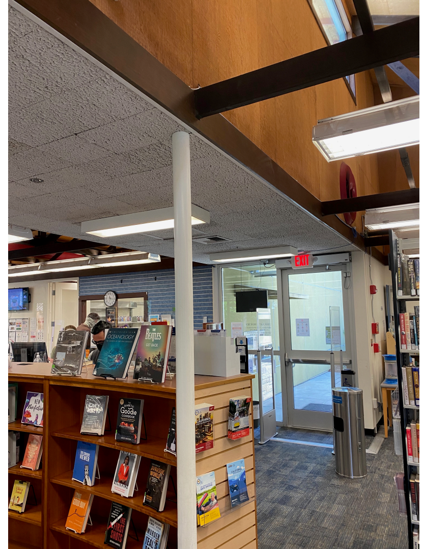
8 foot high ceiling section – right side
