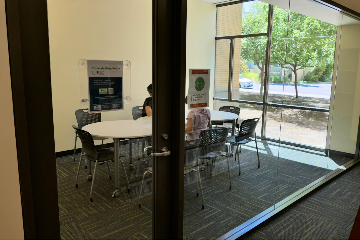
Glass panels connected with caulking
