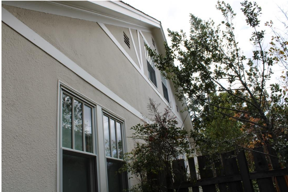
Figure 37. West elevation, facing southeast.
