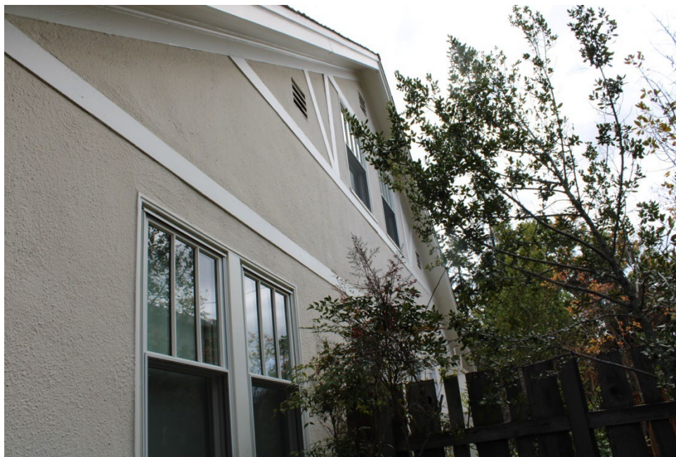
Figure 9. West elevation, facing southeast.
