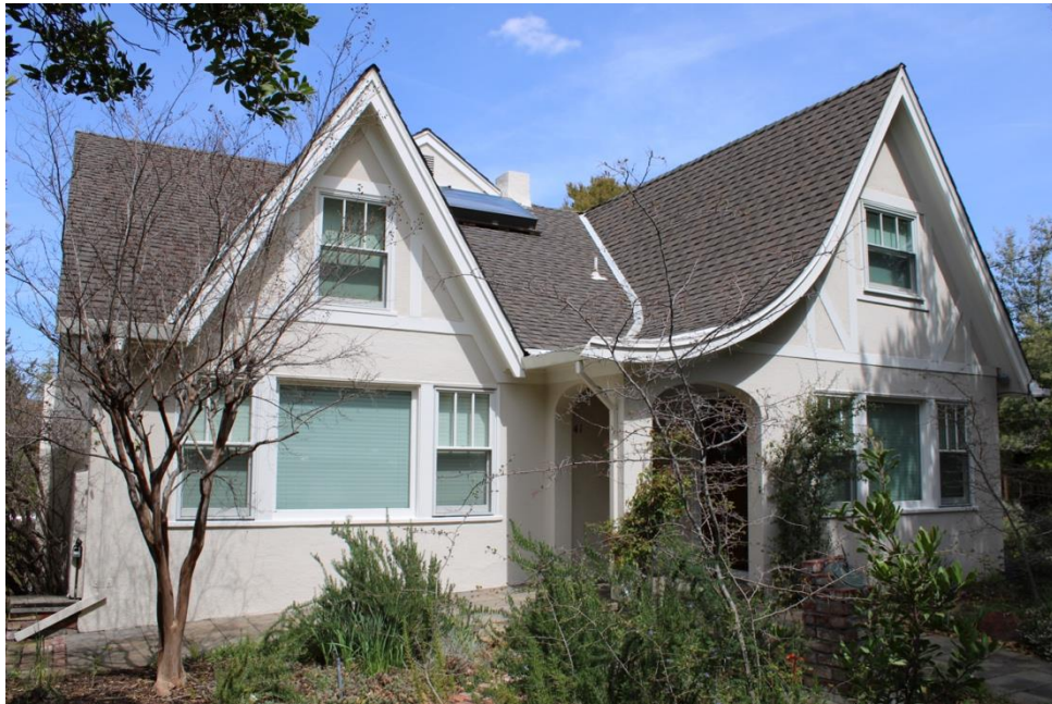
Figure 30. South elevation, facing northeast.
