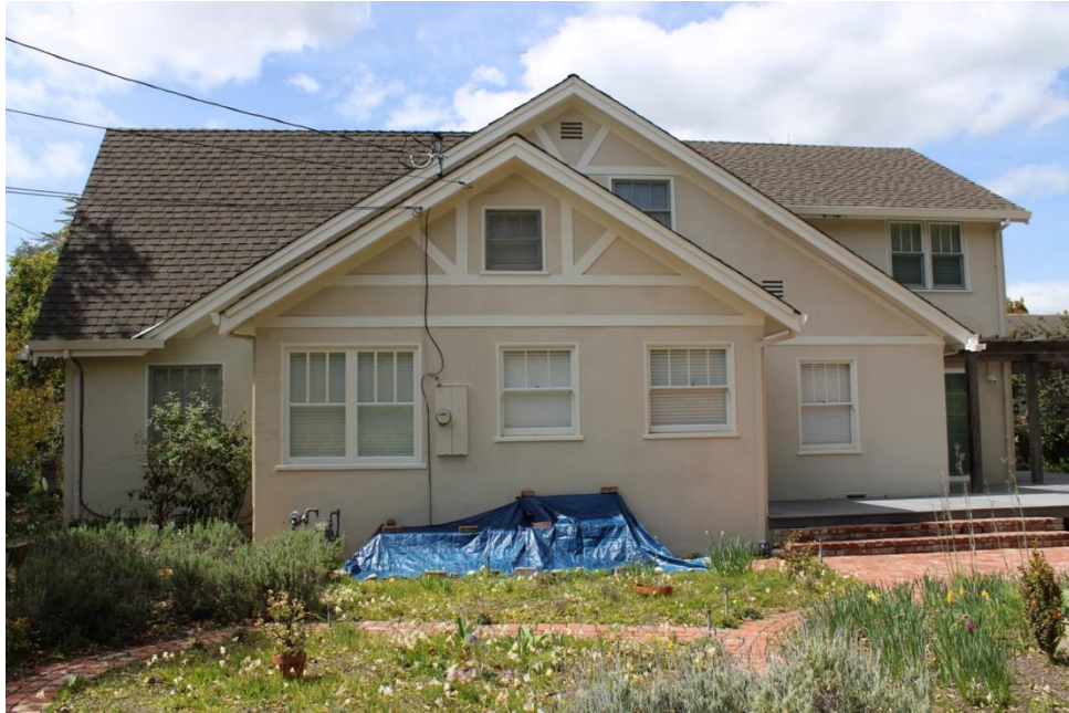
Figure 32. East elevation, facing west.
