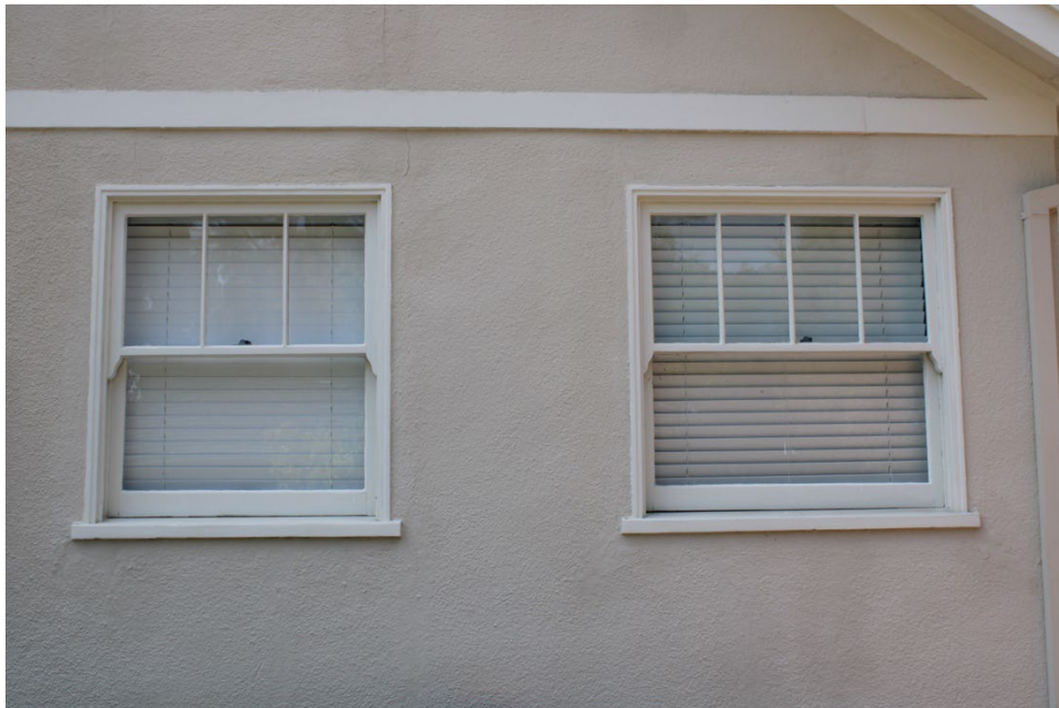
Figure 5. Three-over-one windows with horned stiles (aka lugs) on the east elevation, facing west.
