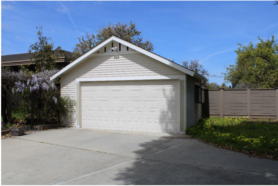
Figure 11. South elevation of detached garage, facing north.
