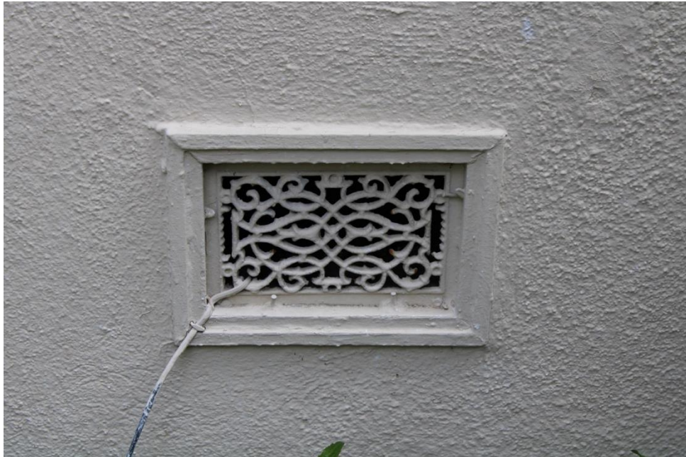
Figure 38. Cast-iron vent cover at the foundation.
