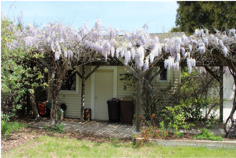
Figure 12. West elevation and trellis-covered walkway, facing east.
