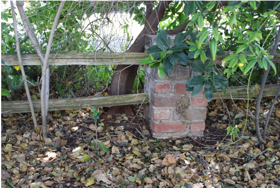
Figure 14. Fence with brick posts and wood rails along southern perimeter of the property.
