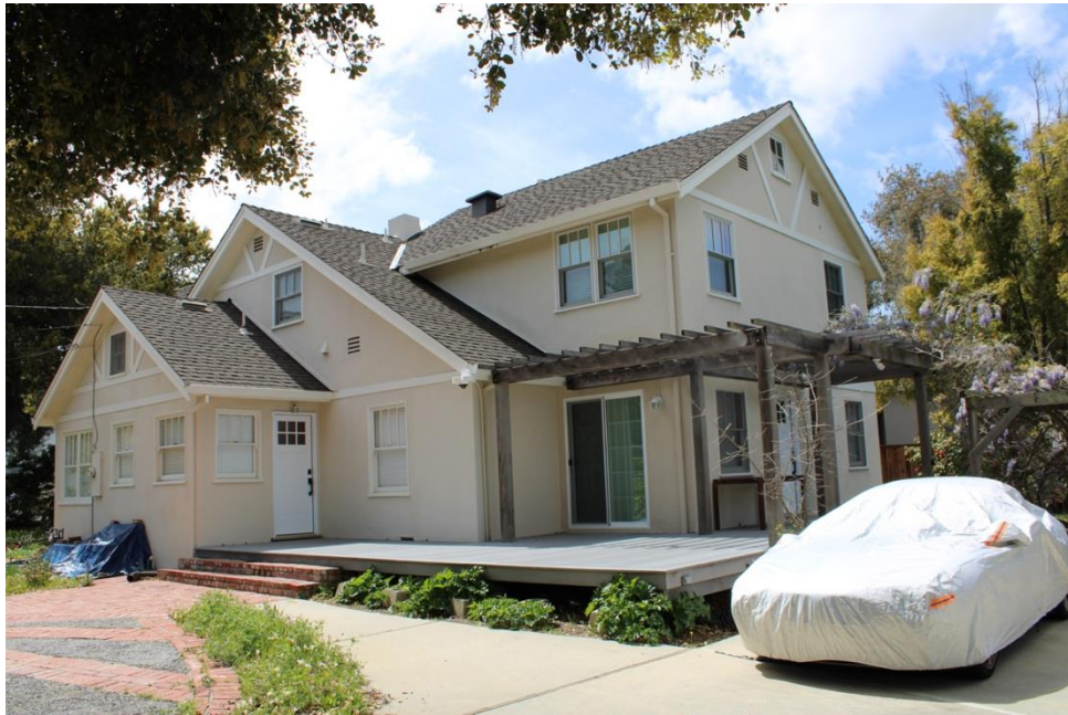
Figure 34. East elevation, facing southwest.
