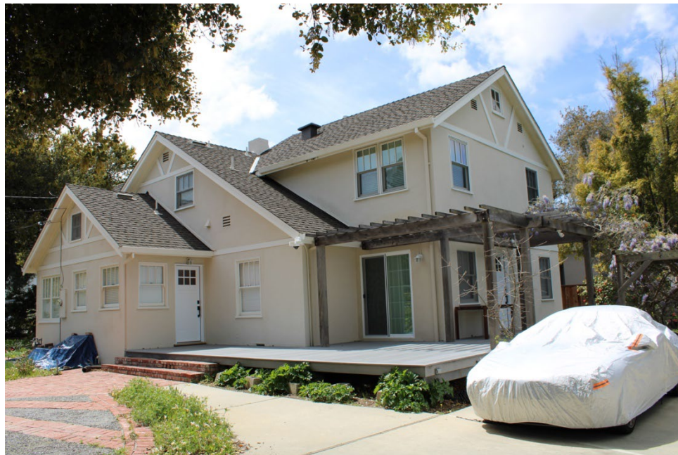
Figure 6. East elevation, facing southwest.
