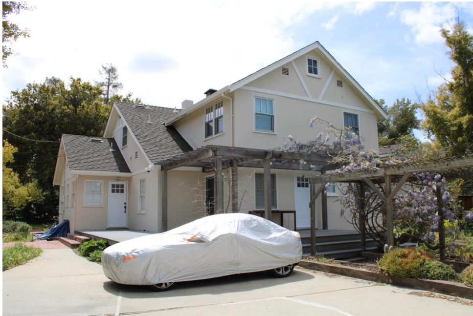
Figure 35. North elevation, facing south.
