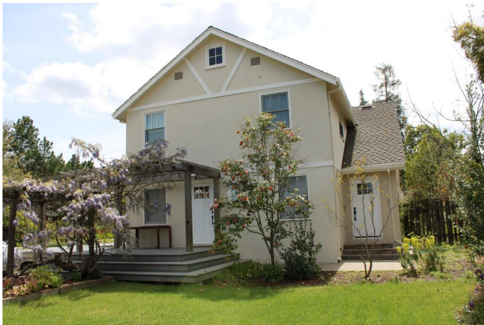
Figure 36. North elevation, facing south.
