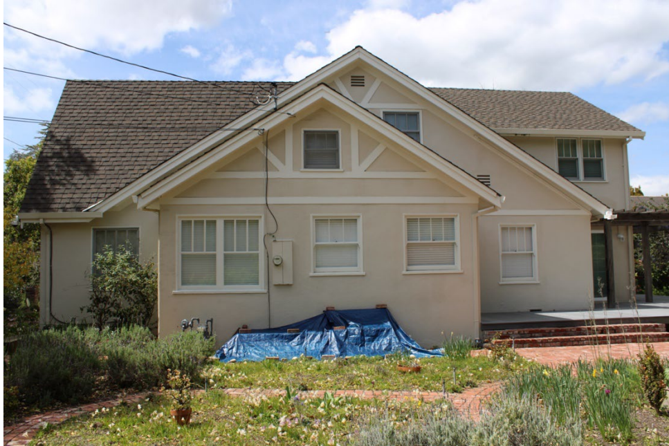
Figure 4. East elevation, facing west.
