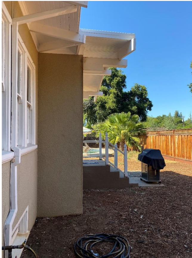
Figure 27. East elevation, facing north.
