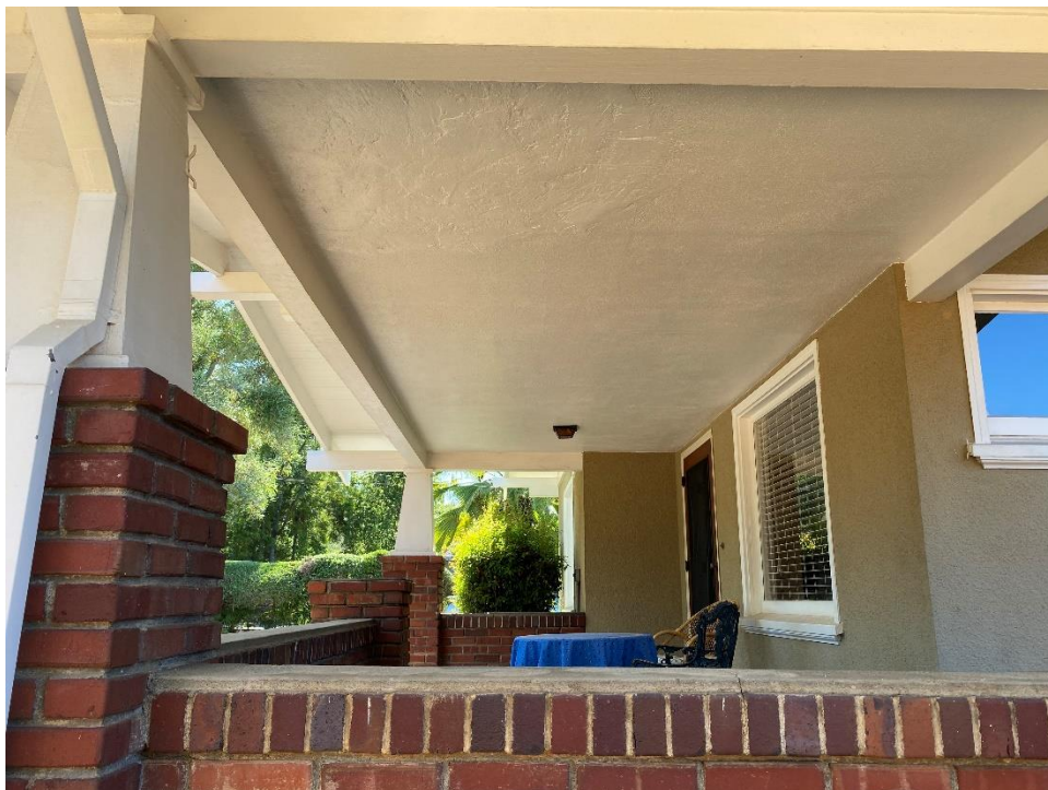
Figure 25. Photograph showing the front porch, facing west.
