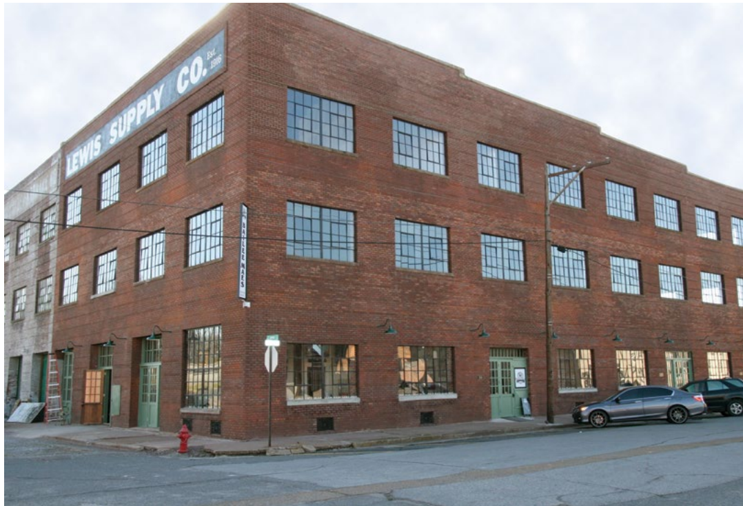
[20 a-d] The original steel windows in this industrial building were successfully repaired as part of the rehabilitation project (left).
