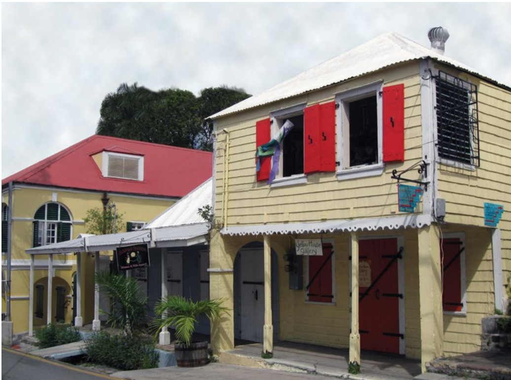
[46] The varied size, shapes, and architectural styles of these historic buildings are unique to this street in Christiansted, St. Croix, USVI, and should be retained in a rehabilitation project.
