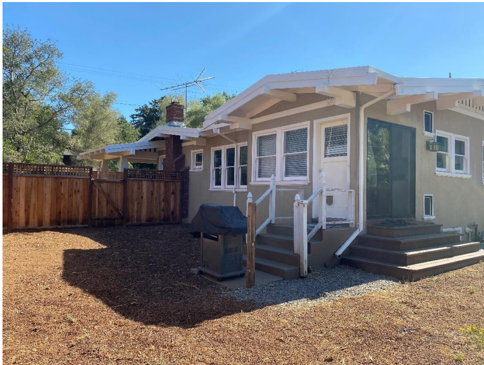
Figure 28. Photograph showing the east elevation, facing southwest.
