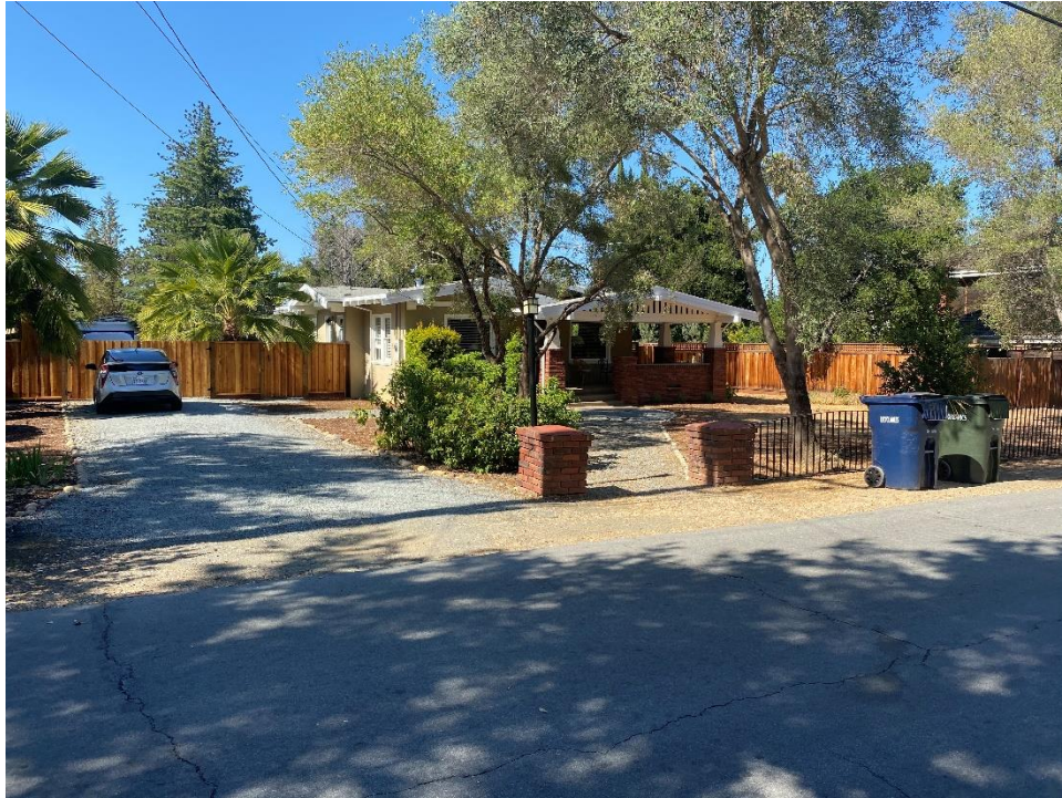
Figure 22. South elevation, facing north.
