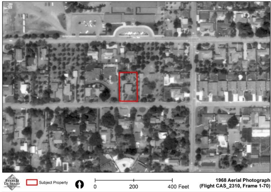
Figure 20. 1968 aerial photograph of the Property with dense residential development around it (courtesy of University of Santa Barbara Library).
