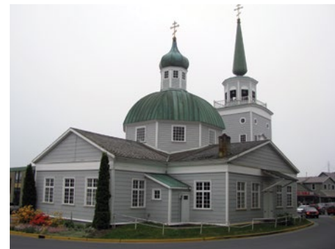
[3] The Cathedral of Saint Michael the Archangel, built in the early 1840s in Sitka, AK, was devastated by fire in 1966. It was reconstructed using measured drawings done in 1961 by the Historic American Buildings Survey (HABS). While the original cathedral was built of logs covered on the exterior with wood siding, its replacement is a fire-resistant structure with concrete and steel walls that replicates the historic building's appearance. Photo: Barek at Wikimedia Commons.
