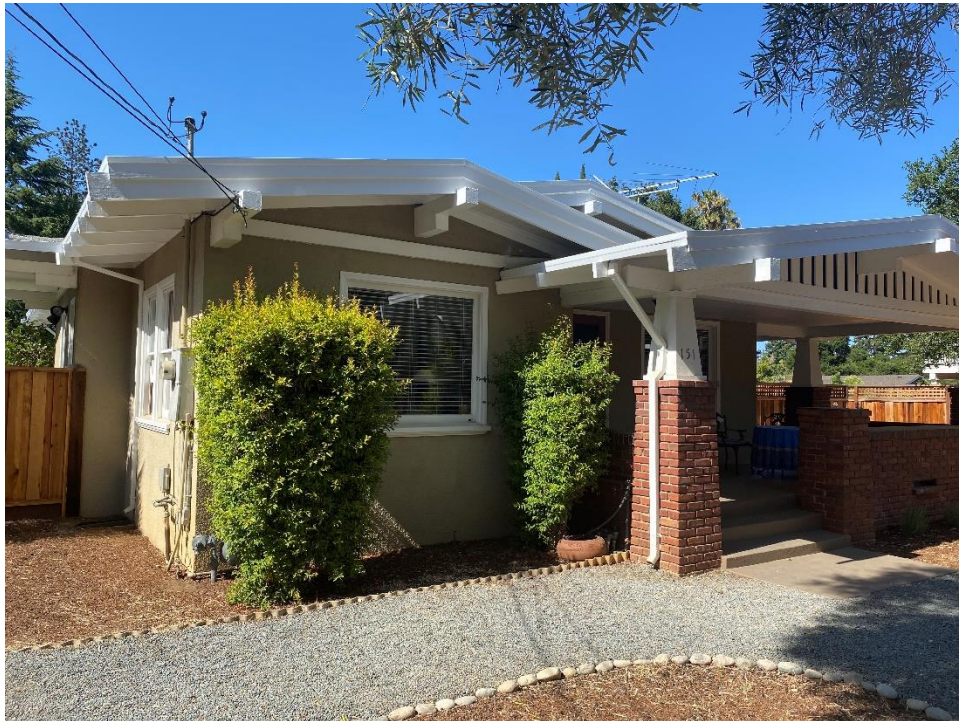
Figure 24. South elevation, facing north.
