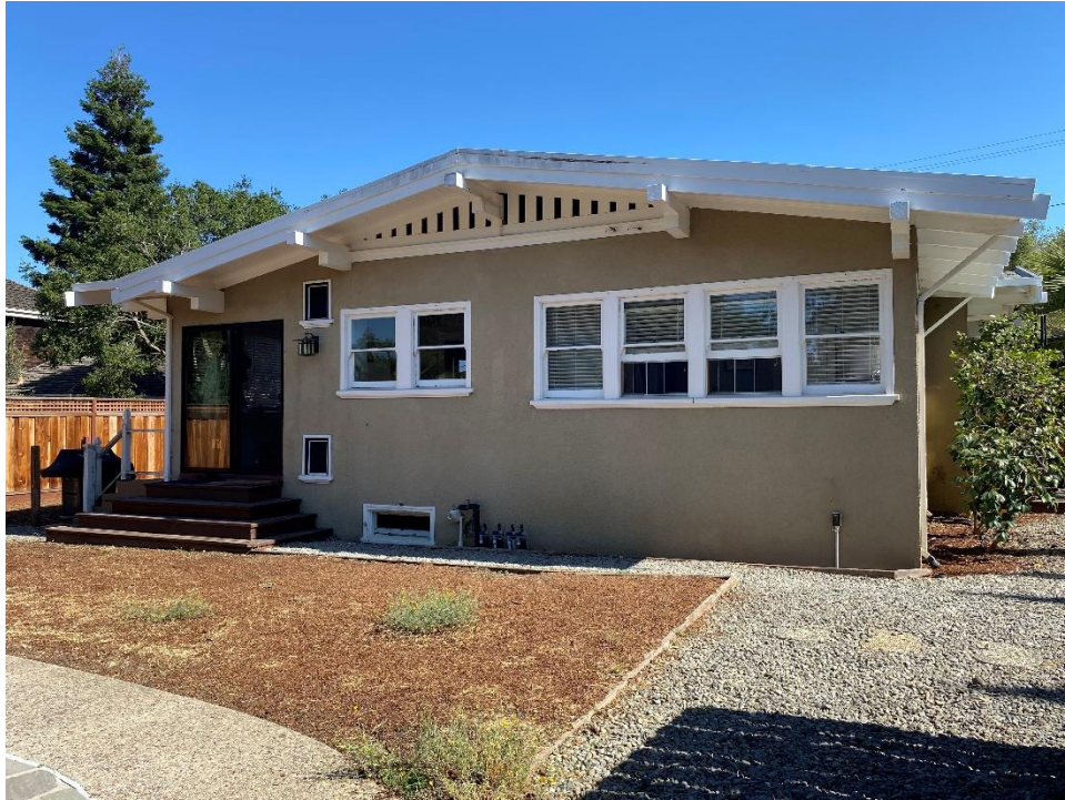
Figure 30. North elevation, facing south.
