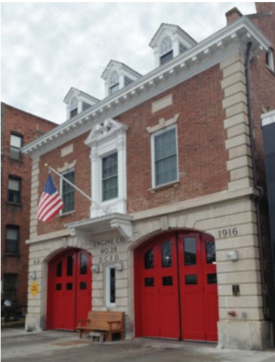
[56 a-b] In order to continue in its historic use, the door openings of this 1916 Colonial Revival-style fire station had to be widened to accommodate the larger size of modern fire trucks. Although this resulted in some change to the arched door surrounds, it is minimal and does not negatively impact the historic character of the building. (a) Above, before; Photo: Fire and Emergency Medical Services Department (FEMS), Washington, D.C.; below, after.
