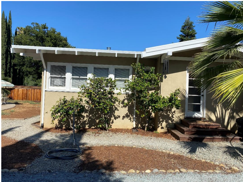
Figure 32. West elevation, facing east.
