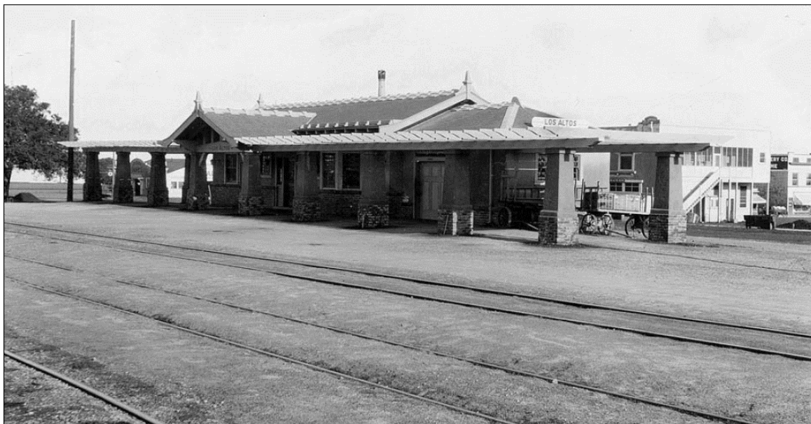
Figure 7. ca. 1920 photograph of the 1913 Southern Pacific Railroad depot in Los Altos (courtesy of the Los Altos History House Museum Archives).
