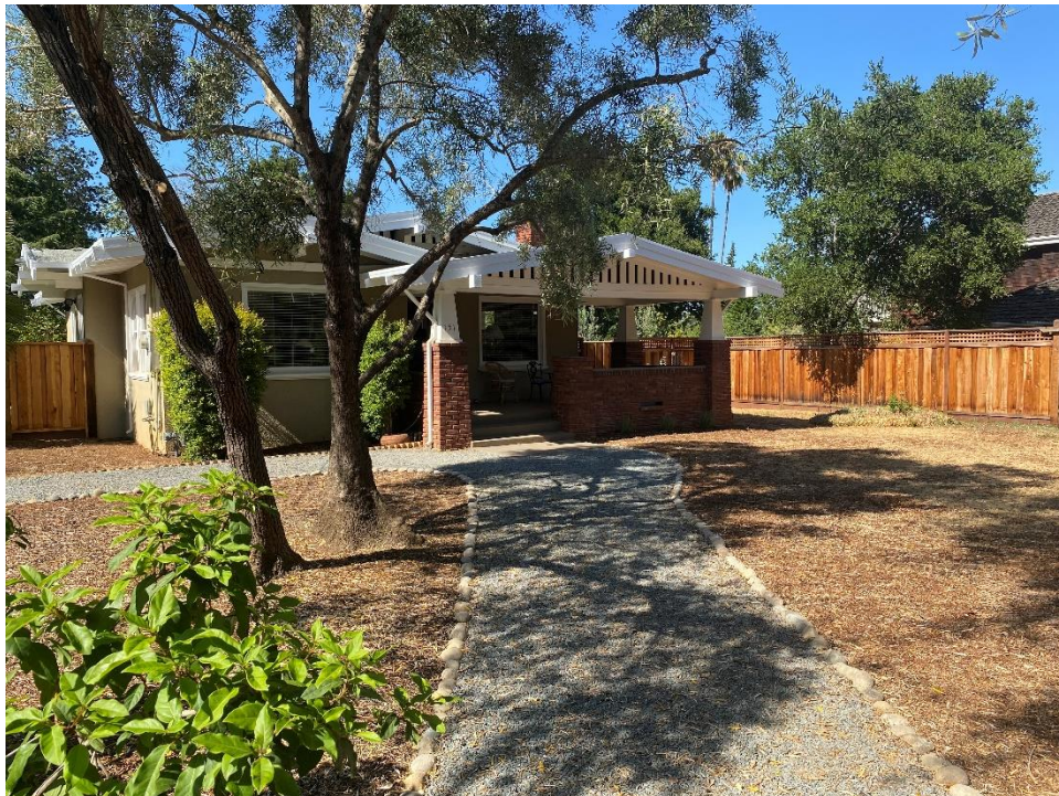
Figure 23. South elevation, facing north.
