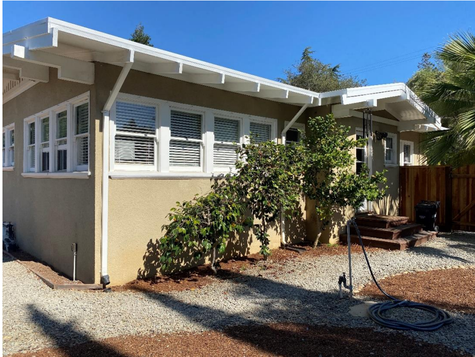
Figure 31. West elevation, facing southeast.
