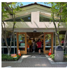
Existing Library Main Entrance
