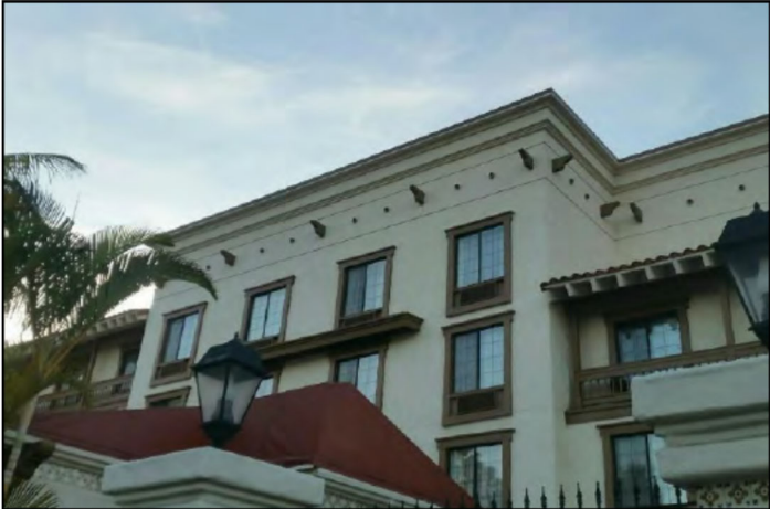
Figure 2: This completely concealed wireless telecommunications facility, including antennas, is cited in the City of San Diego's Land Development Manual in its guidelines for wireless communications facilities.
