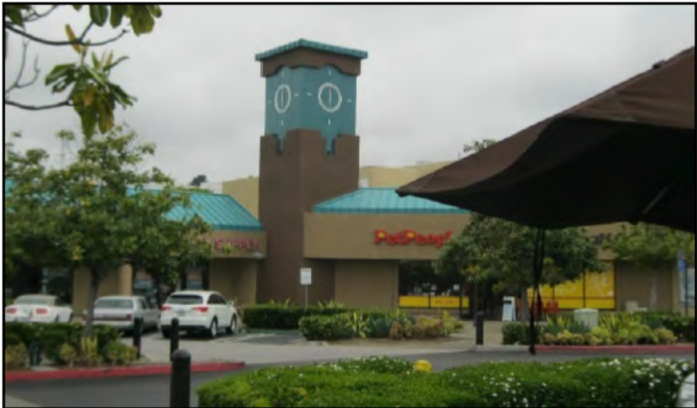
Figure 4: A cupola (above) and a clock tower (below) conceal antennas.
