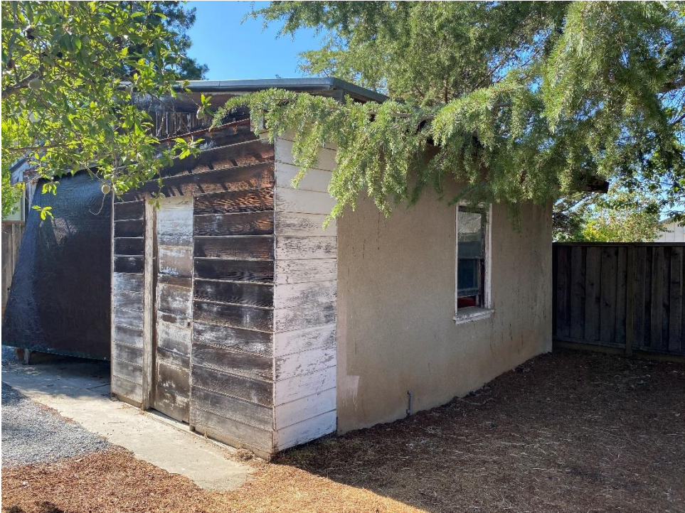
Figure 33. Photograph showing the cladding along south and east elevations, facing northwest.
