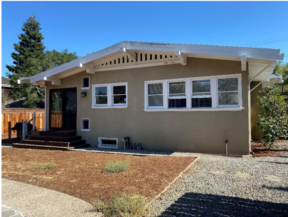
Figure 30. North elevation, facing south.
