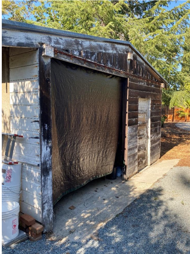
Figure 34. Photograph showing the tarp covering the wide door opening and the front entrance to the shed.
