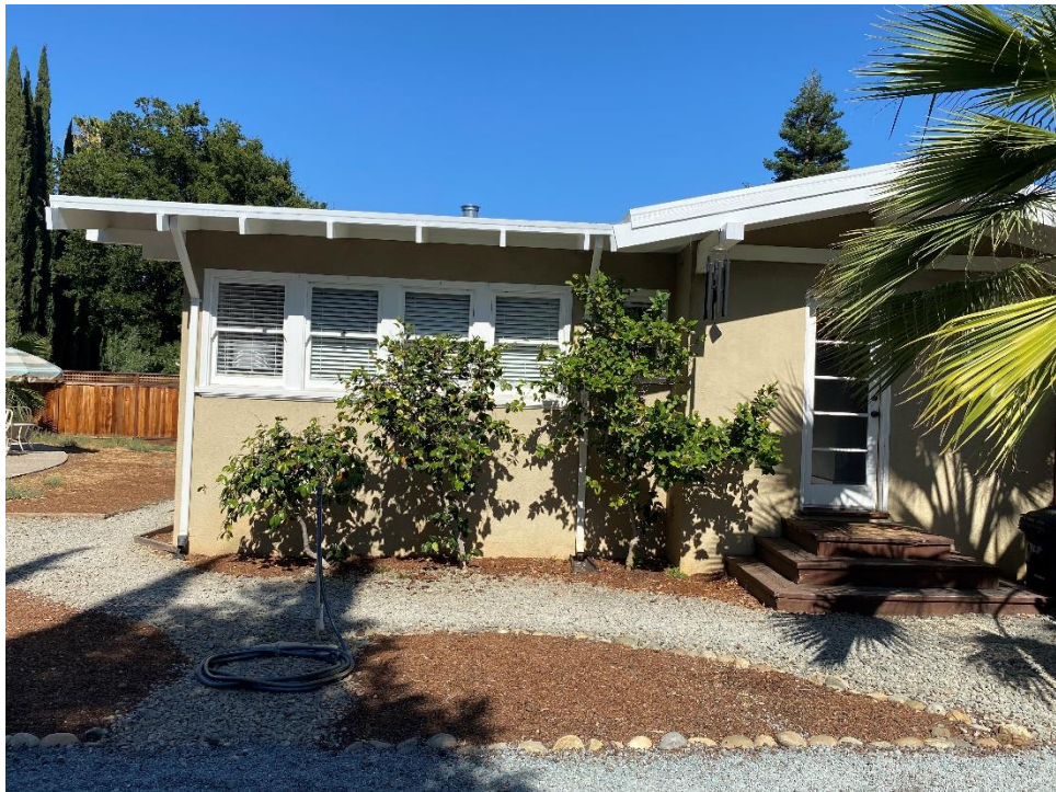
Figure 32. West elevation, facing east.
