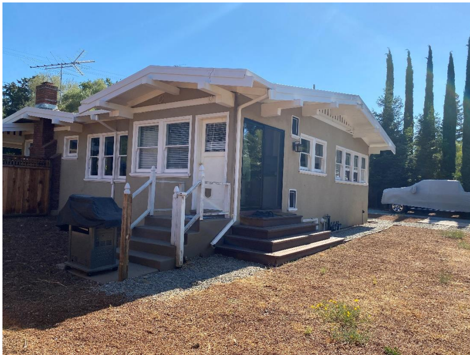
Figure 29. Photograph showing the north elevation rear roof gable and decorative vertical wood boards along the gable, facing southwest.
