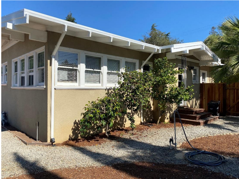
Figure 31. West elevation, facing southeast.
