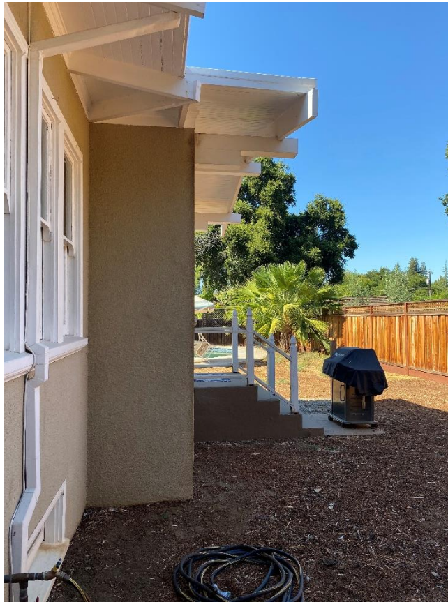
Figure 27. East elevation, facing north.
