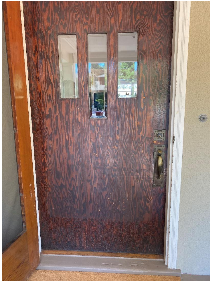
Figure 26. Photograph showing the front door, facing north.
