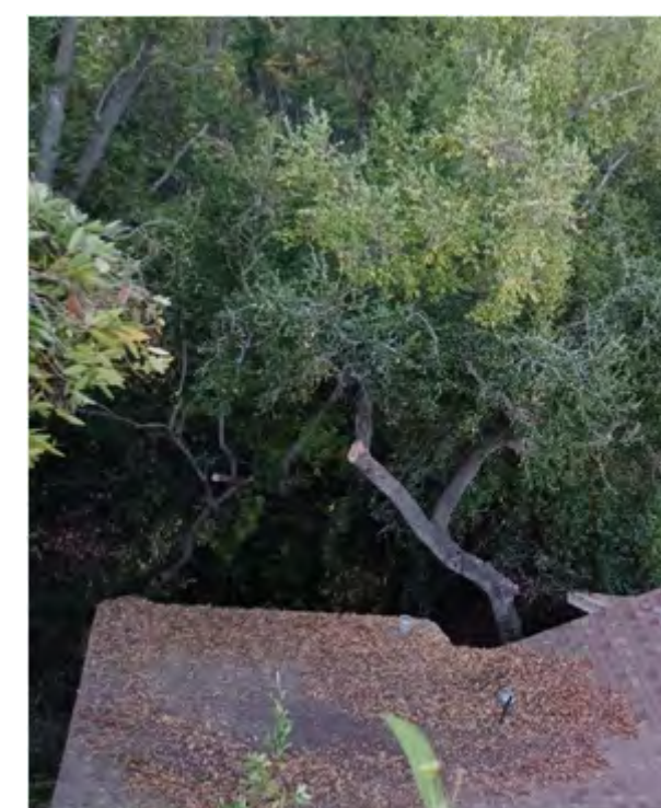
Clearance to Cottage (Tree 7, 8)
