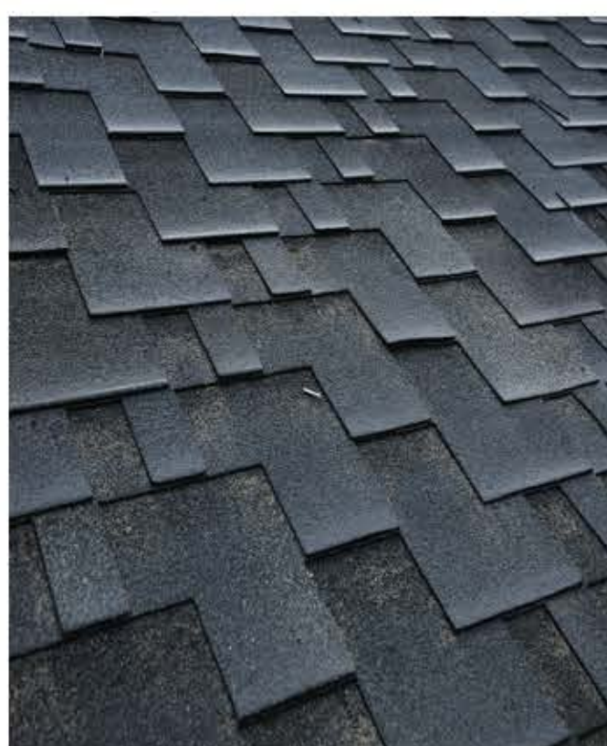
ROOFS ASPHALTIC SHINGLE - MAIN ROOF
