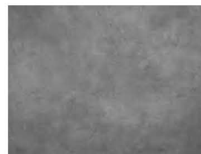
CONCRETE - GARAGE & OTHER AREAS
