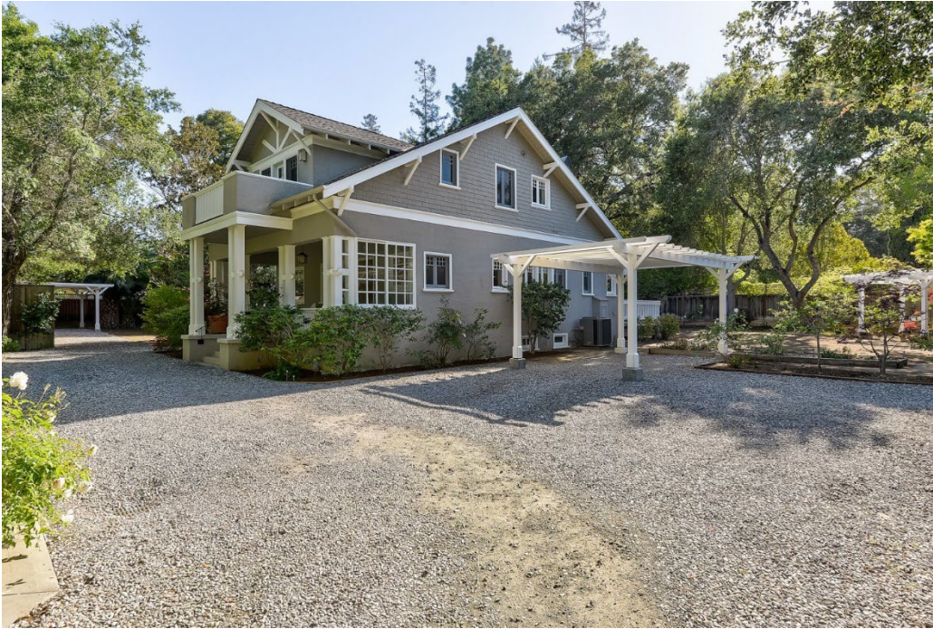
Photograph 4 236 Eleanor Avenue, Los Altos View: The north side façade showing the window alteration to fill the side of the porch and the second level gable. A carport is under the pergola structure and the entrance to the rear of the house..
