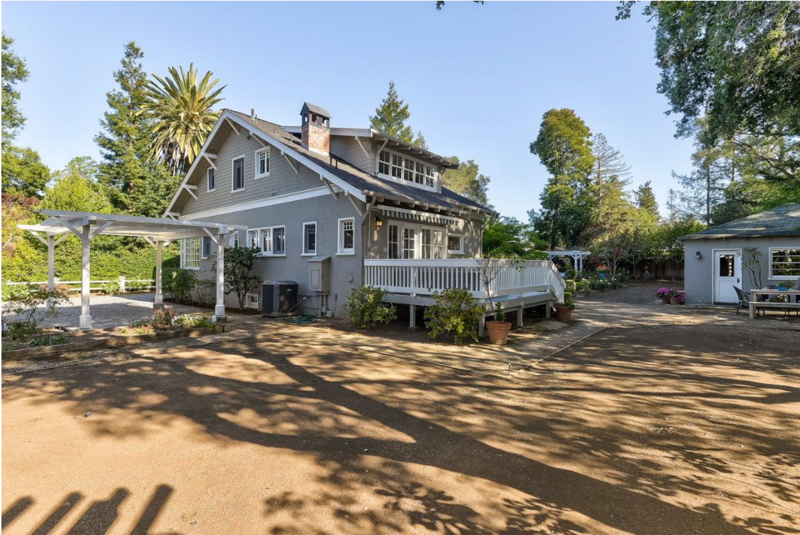
Photograph 6 236 Eleanor Avenue, Los Altos View: Rear and north side showing the rear additions and deck addition. A shed is behind the house and the carport on the left (north ) side.
