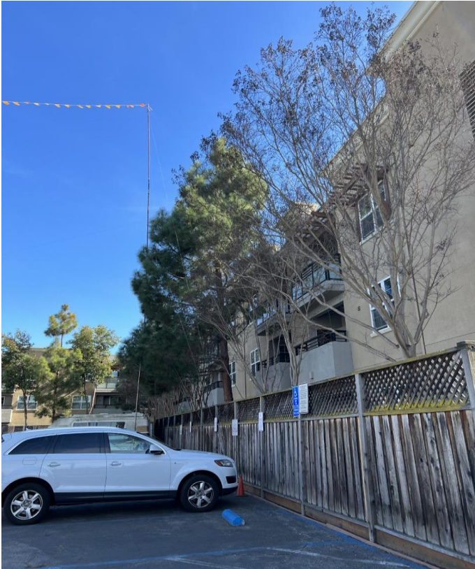
Picture 1 (South Side Bldg Property Line Pole)
