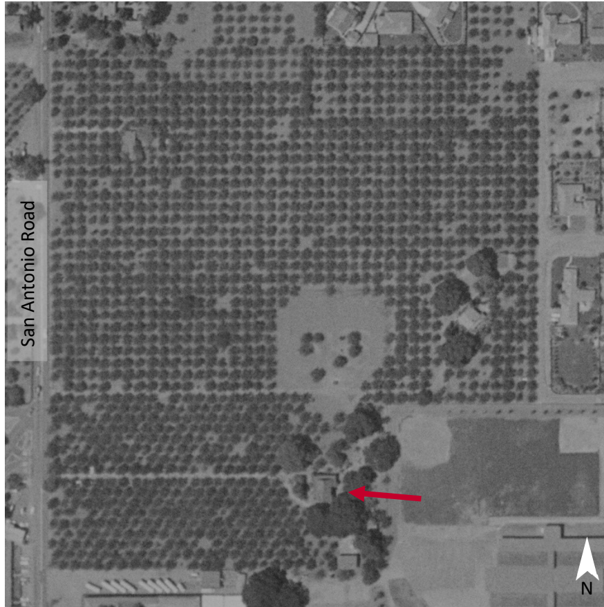
Figure 14. 1956 aerial photograph of the general area of the orchard, Smith House is identified with a red arrow.
