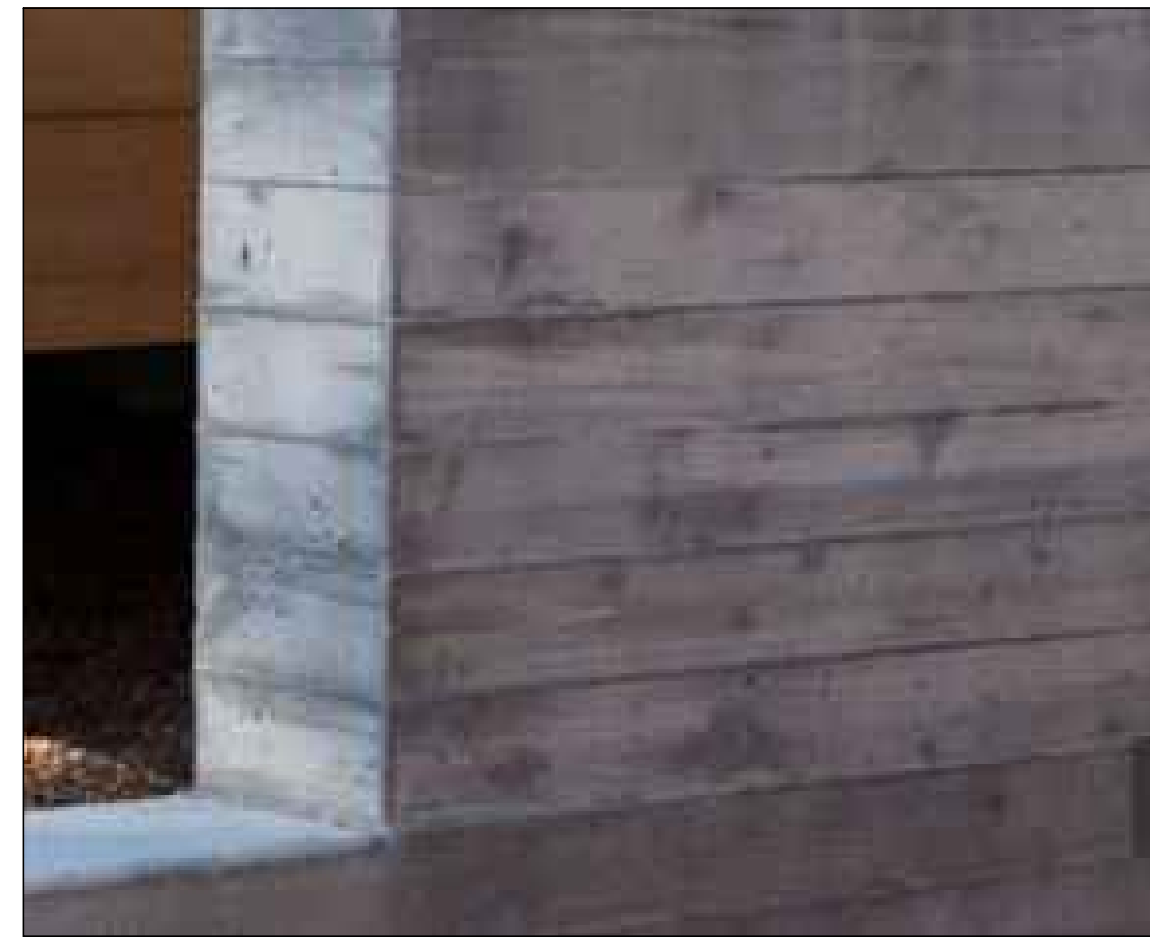
BOARD FORMED CONCRETE
