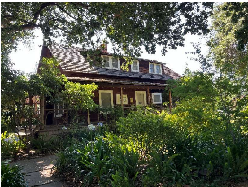
Figure 8. The west façade.
