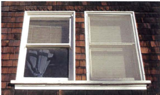
View of the second floor windows at the east elevation. These windows are wood one-over-one light, double hung sash in good condition. The windows will remain, but they will be re-glazed with laminated glass without a tint.
