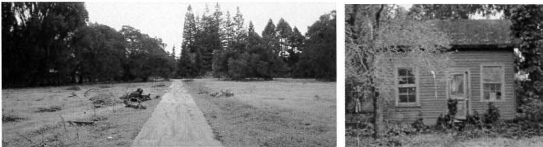
View looking down the asphalt-clad rosary walk at the Corpus Christi Monastery, evaluated for the Menlo Park environmental assessment (left). The building at the right above is single wall construction house, probably dating to the 1850s or early 1860s, on the monastery grounds. This building, which dates to the founding of Menlo Park, was not documented prior to this environmental assessment.
