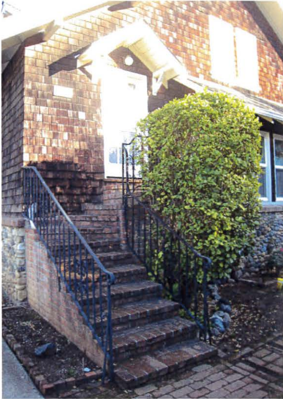
View of the brick exterior stair at the south side of the east elevation.
