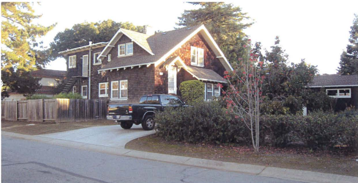
View of the south and east exterior walls of the house facing northwest. The garage/in-law unit is at the right. The chimney, discussed immediately above, is proposed for removal.
