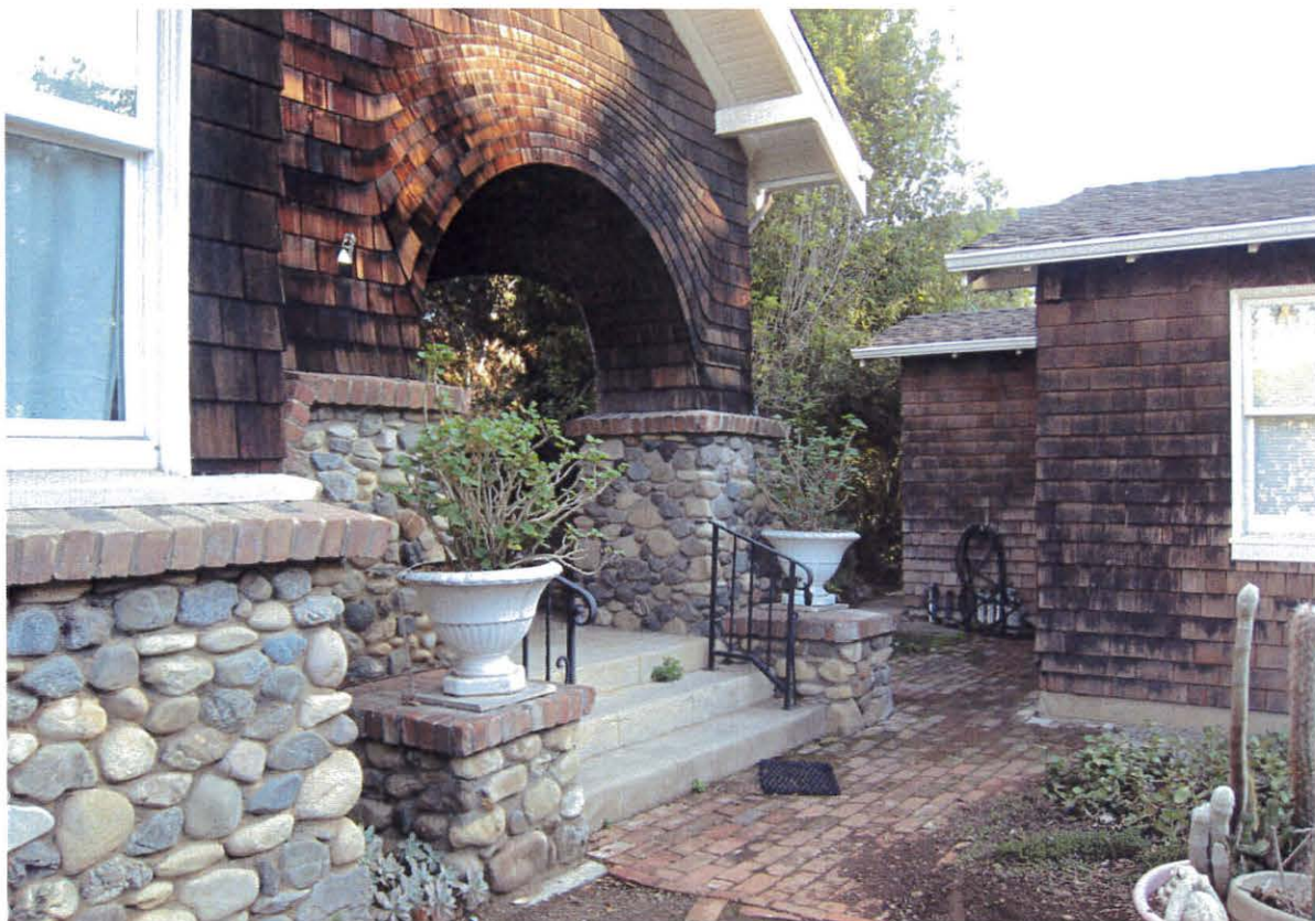
View of the house at the left and the garage/in-law unit at the right.
