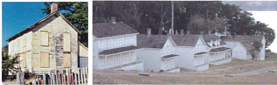
View of the Carrington Ranch House (left) and Officers Row (right).
