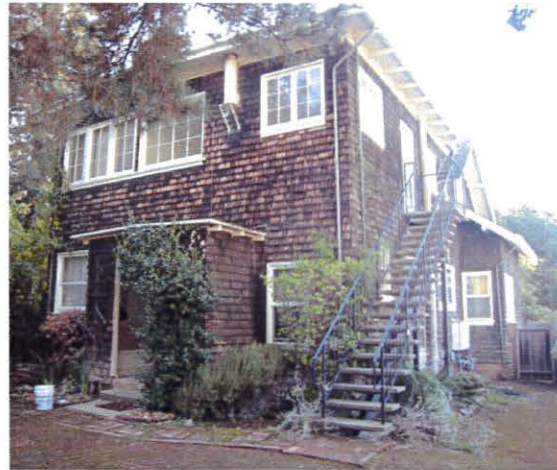
View of the west or rear elevation. Although this elevation is visible from Miravalle Avenue, the owner is proposing to replace all of the second floor windows with double-glazed, wood casement sash with interior and exterior grids to suggest the light configuration of the existing. The 12-light sash shown above is a fixed (inoperable) window; it is proposed for replacement with operable casement windows. The exterior staircase at the right will remain.
