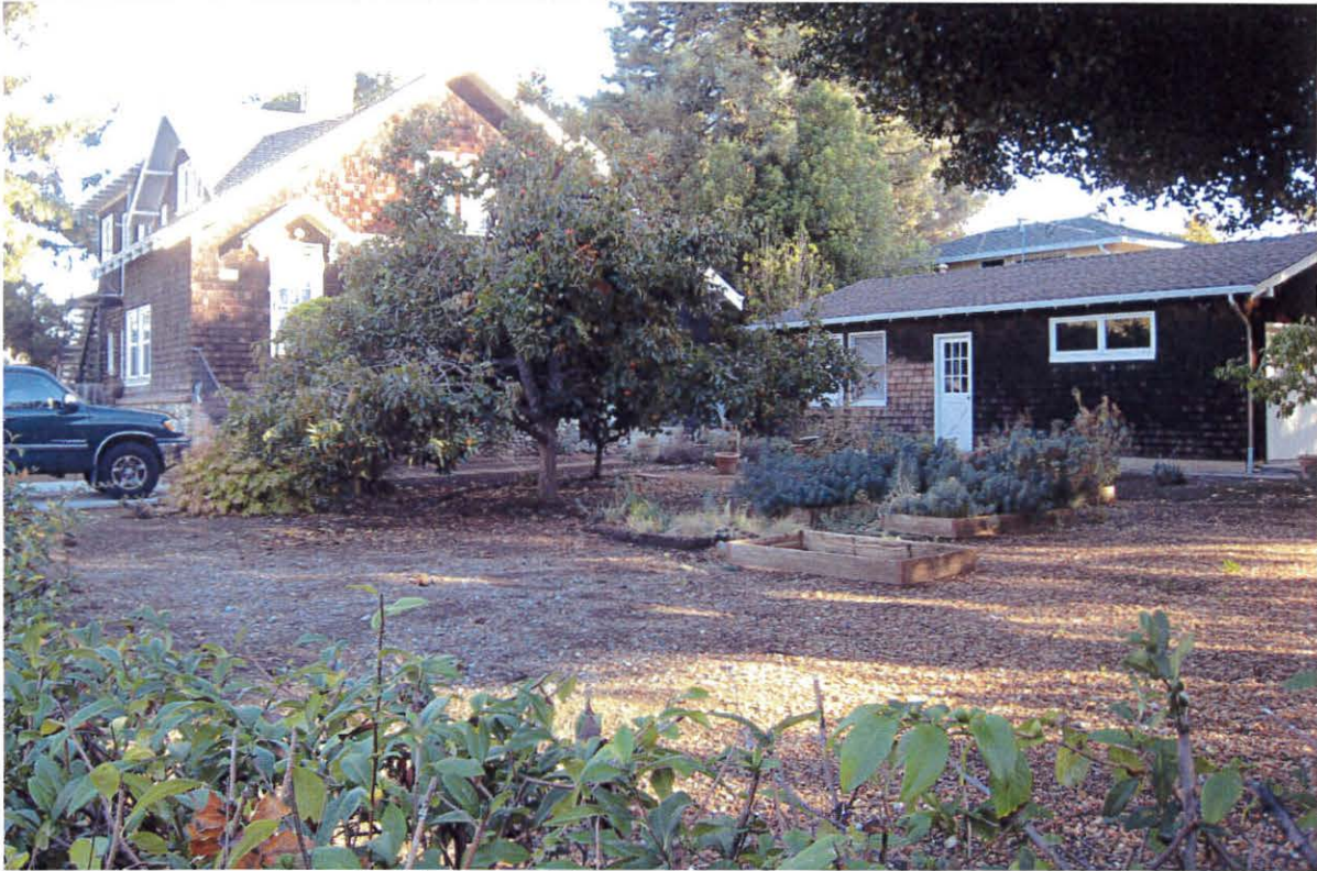
View of the east exterior wall of the house facing northwest. The garage/in-law unit is at the right.
