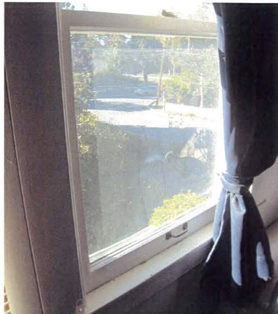
Interior view of the same windows.
