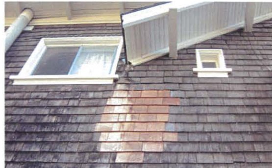
The windows at the left are non-historic sash which will be replaced with double-glazed, wood casement sash with interior and exterior grids to suggest the same light configuration as the adjacent historic windows. The small window at the right is the third and final small window proposed for removal.
