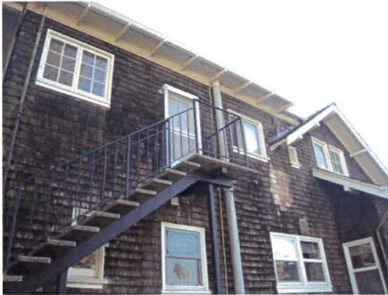
View of the window openings in the west exterior wall.
