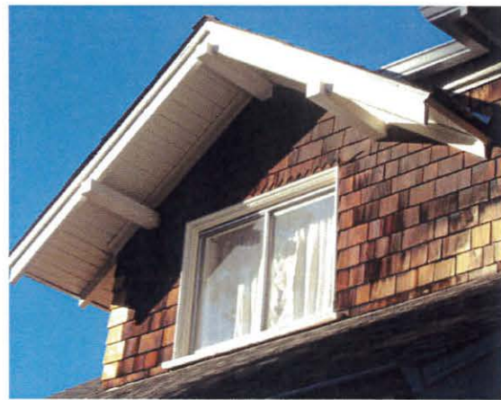
View of the easternmost windows at the second floor. These windows are not original nor are they considered historic. The windows will be replaced with double glazed wood casement sash with applied exterior and interior grids to suggest four lights per leaf. Please see window cut sheets incorporated into the drawings. The drawings show a new window to the right of the above window; it will be similar to the new sash proposed for the above opening, but double hung.
