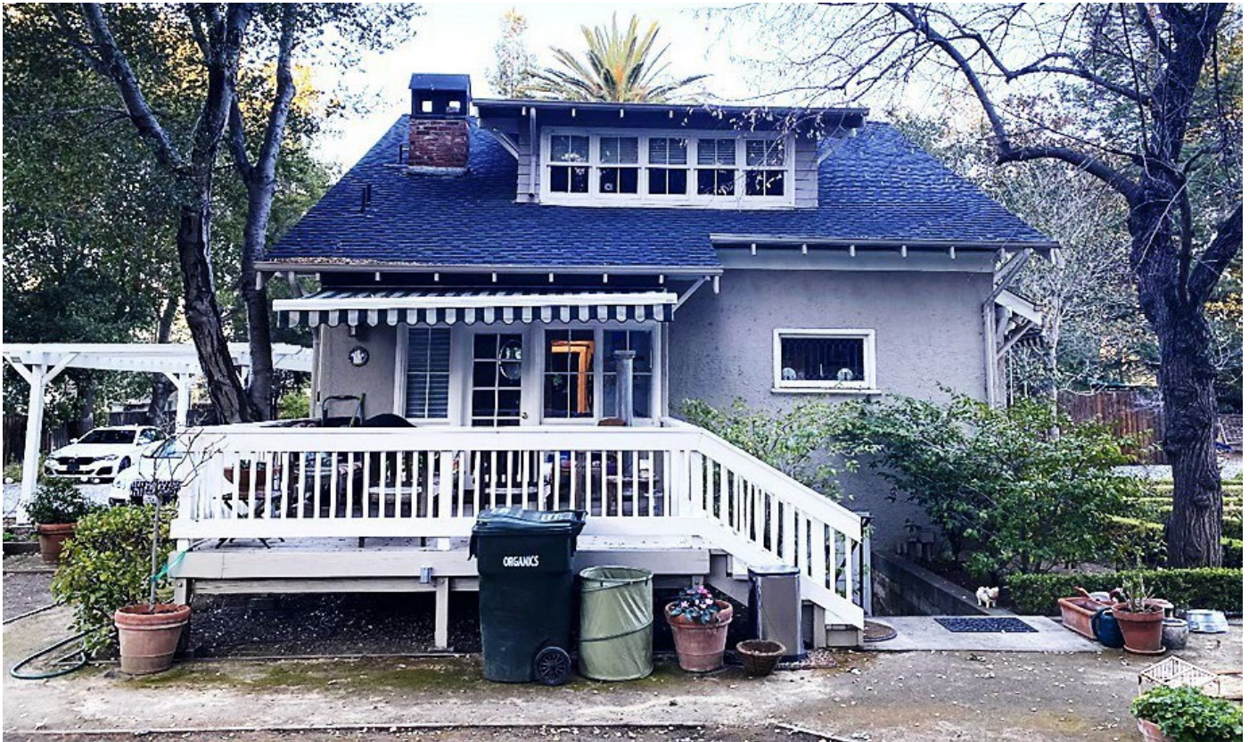
Photograph 7 236 Eleanor Avenue, Los Altos
