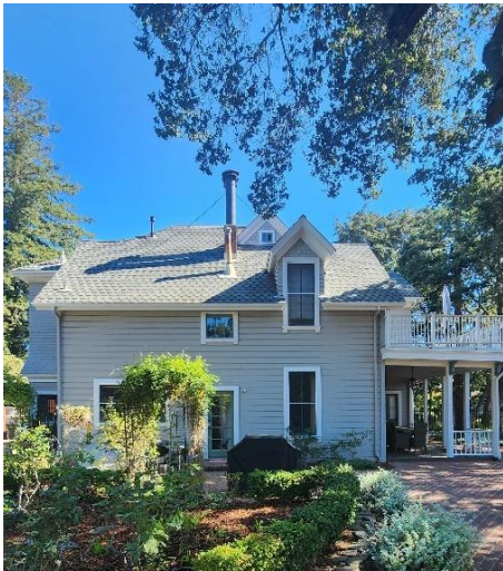
Existing west facade
