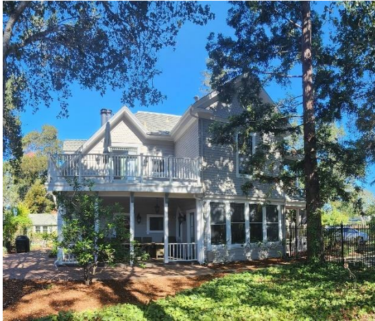
Existing south facade
