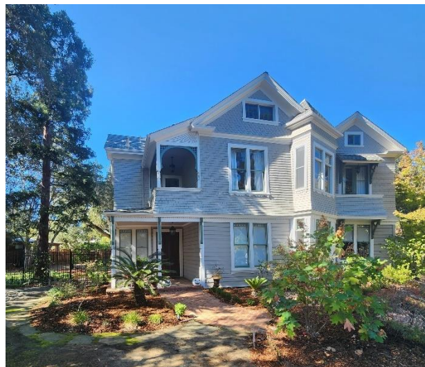
Existing east facade
