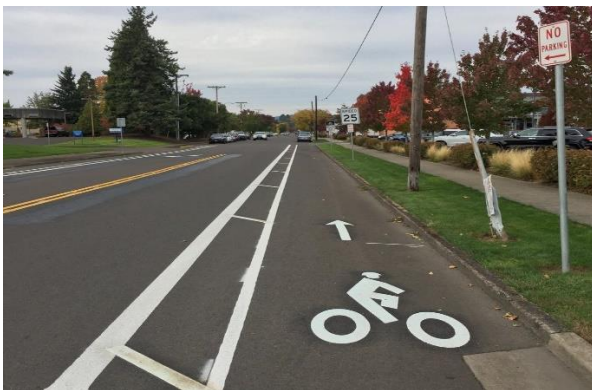
Buffered Bike Lane (Class IIB) – Striping only
