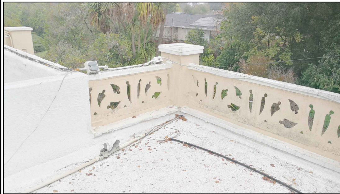
IMAGE C: @ UPPER BALCONY PARAPET
