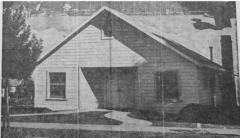
Figure 7. Exterior view with V-groove wood siding, 1941 (Los Altos Newspaper, 1941)
