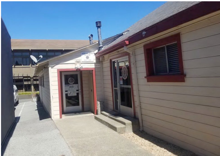
Figure 10. West elevation looking north (W. Bassett, 2021)
