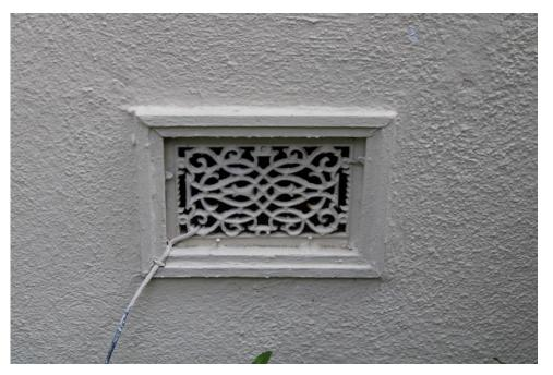
Figure 38. Cast-iron vent cover at the foundation.
