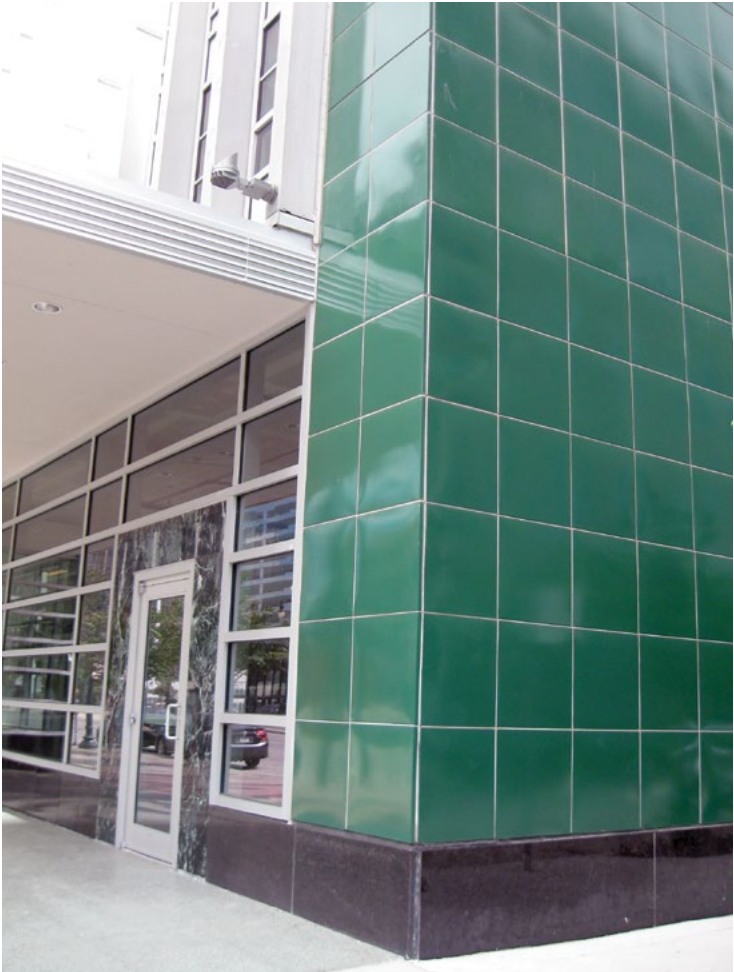
[15] New enameled-metal panels were replicated to replace the original panels, which were too deteriorated to repair, when the storefront of this early 1950s building was recreated.
