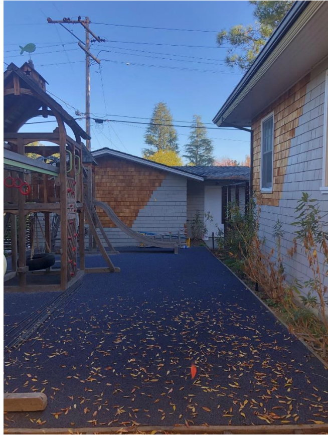
Figure 8 – South (garage – to left, and addition – to right) elevation
