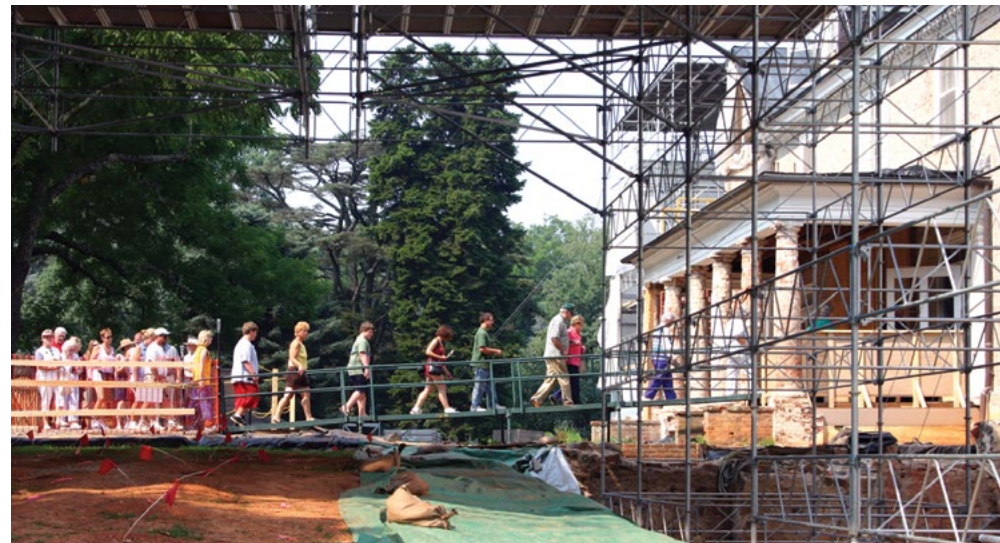
[16] Archeological investigation of the property was undertaken to ensure accuracy of the restoration of Montpelier. Photo: Courtesy of The Montpelier Foundation.
