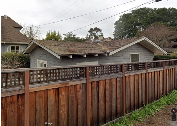
Figure 6 –North (alley side) elevation
