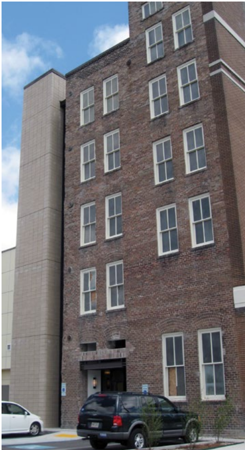
[62] The stair tower at the rear of this commercial building is a compatible new addition.
