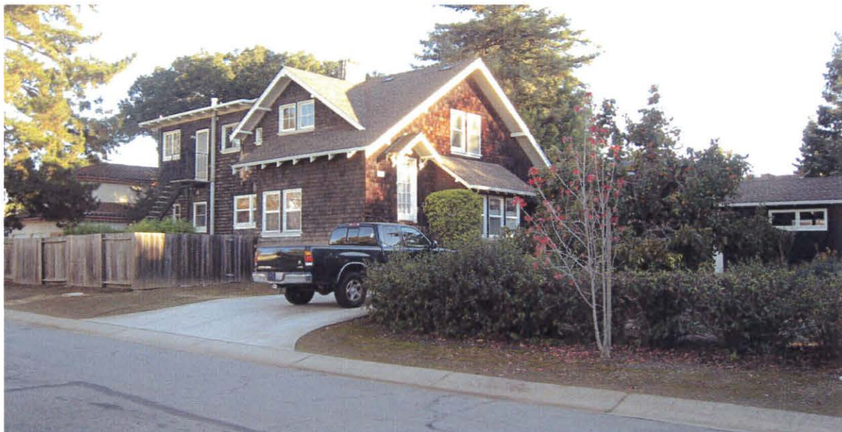
View of the south and east exterior walls of the house facing northwest. The garage/in-law unit is at the right. The chimney, discussed immediately above, is proposed for removal.
