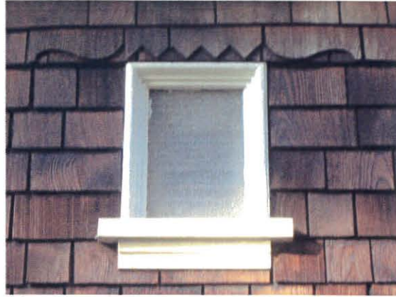
The above window is proposed for removal. It faces the east side garden and is not visible from a public right-of-way.
