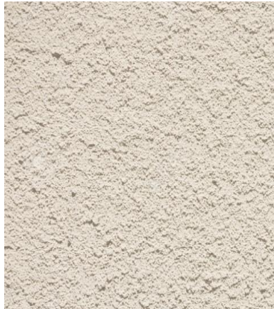
STUCCO WALL FINISH PAINTED WITH KM5759 COLOR
