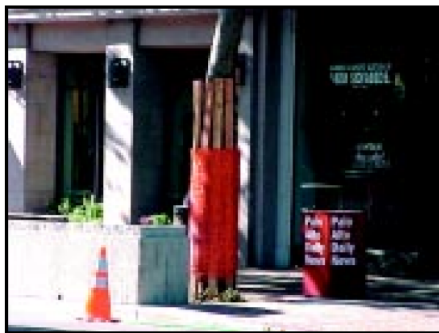
IMAGE 2.15-4 Trunk Wrap Protection
