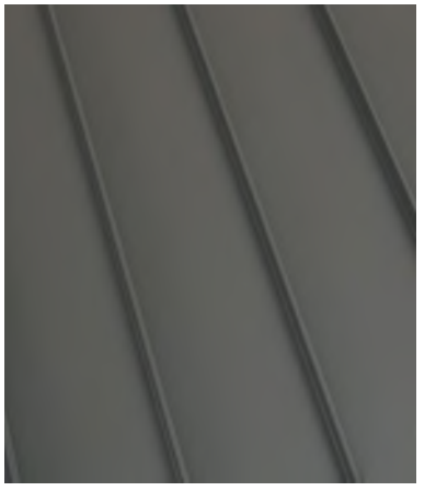
STANDING SEAM METAL ROOF
