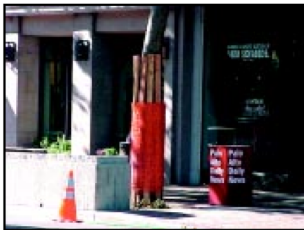
IMAGE 2.15-4 Trunk Wrap Protection
