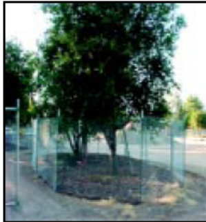
IMAGE 2.15-1 Tree Protection Fence at the Dripline
