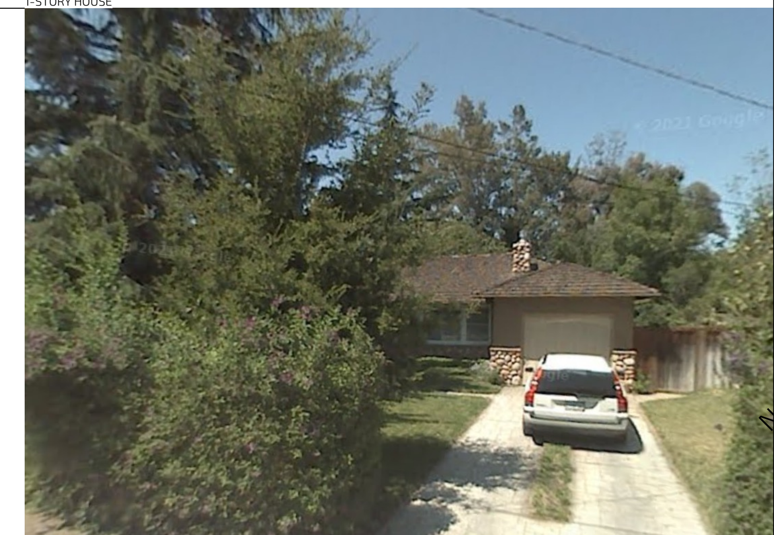
916 SEENA AVE 1-STORY HOUSE
