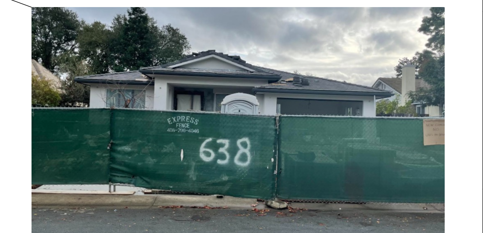
638 BENVENUE AVE (IN CONSTRUCTION) 1-STORY HOUSE
