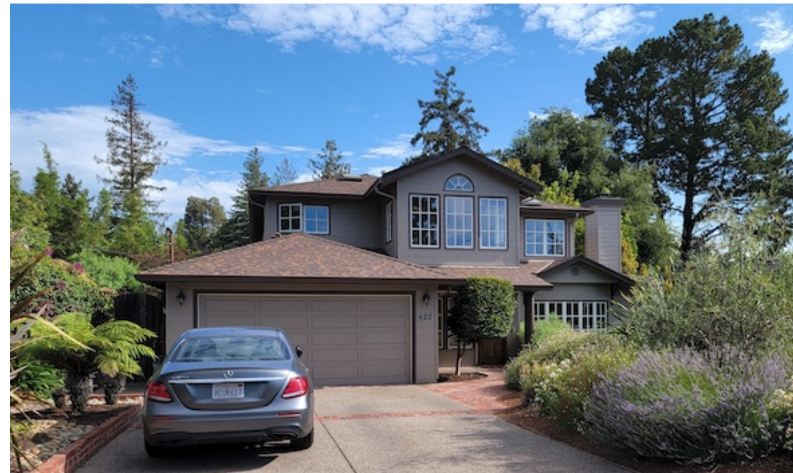
623 BENVENUE AVE 2-STORY HOUSE
