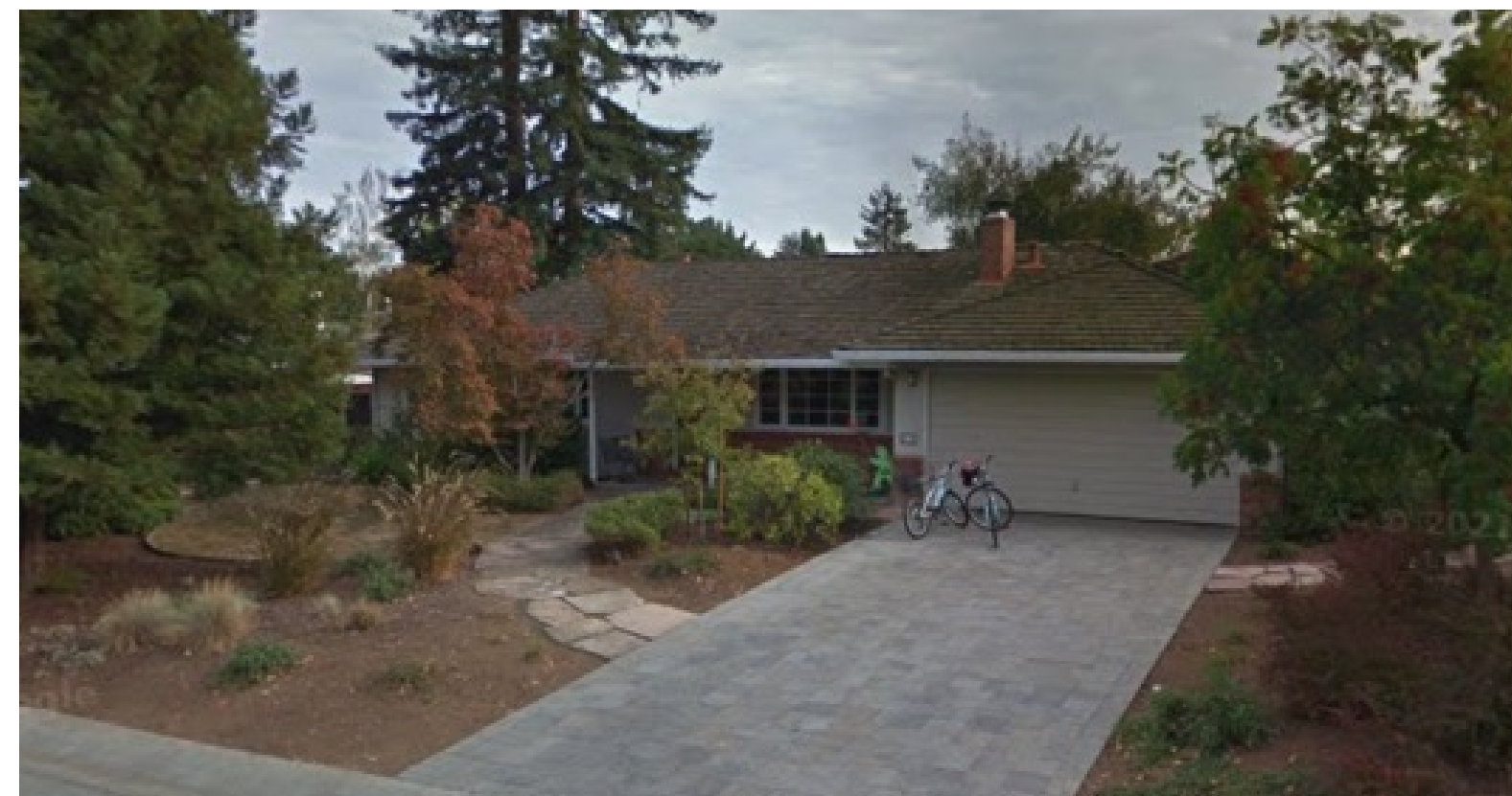
618 BENVENUE AVE 1-STORY HOUSE
