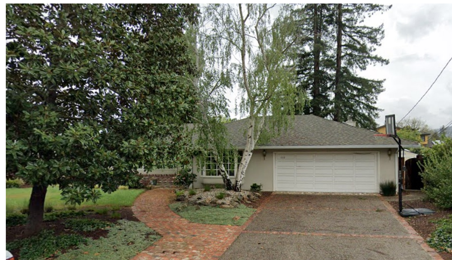
622 BENVENUE AVE 1-STORY HOUSE
