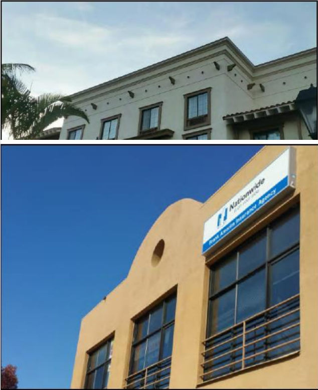
Figure 2: Antennas are concealed behind the circular element.
