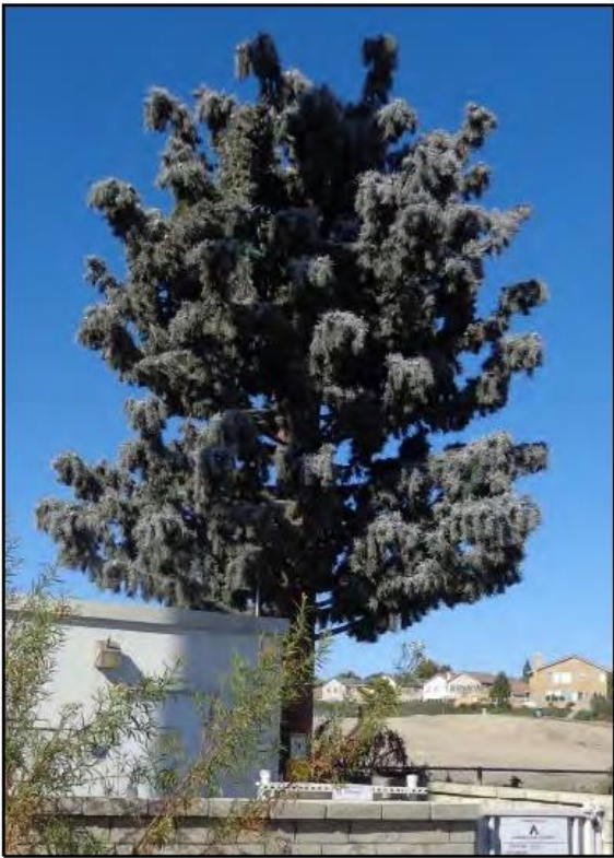
Figure 6: In this example, antennas are concealed by the faux "mono-pine."
