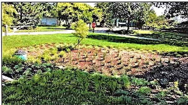
Dry detention pond with planted bottom
