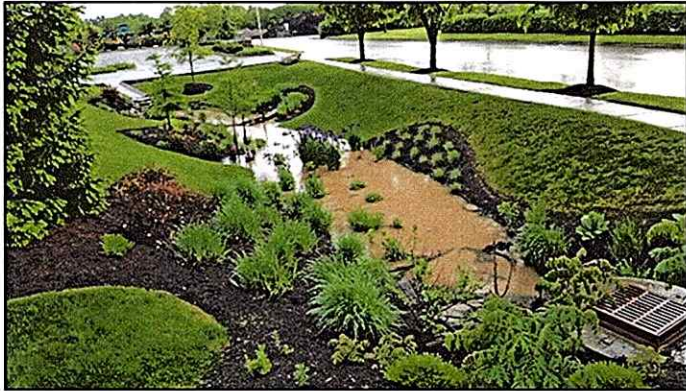
Wet pond in a commercial development acting as a first point of treatment. Note the inclusion of several species of trees and shrubs.
