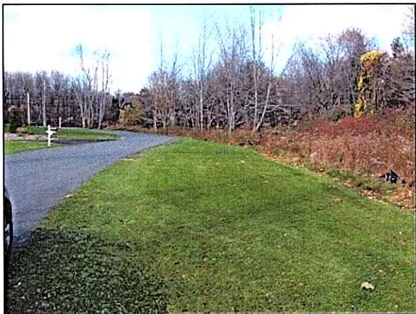
Vegetated filter strip in a residential setting
