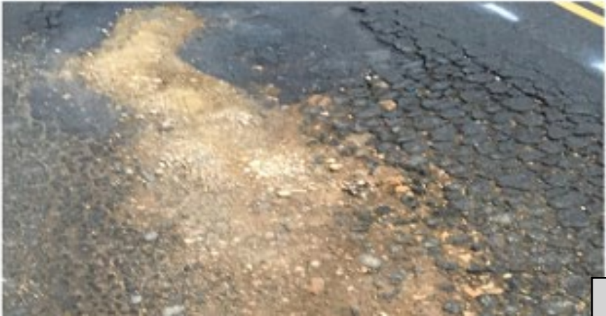
Pavement Condition 0 – 10 (Failed)
