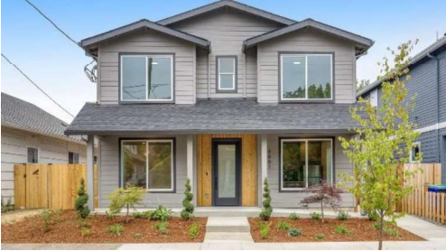
Figure 12. A Newly Built Fourplex in Portland, OR
