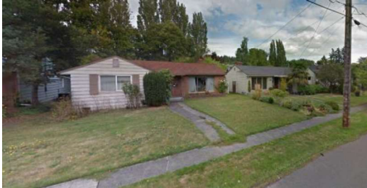
Figure 60. View of Site 4 from NE 170 th Street
