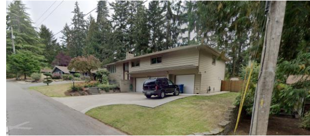
Figure 52. Houses on NE 189 th Place
