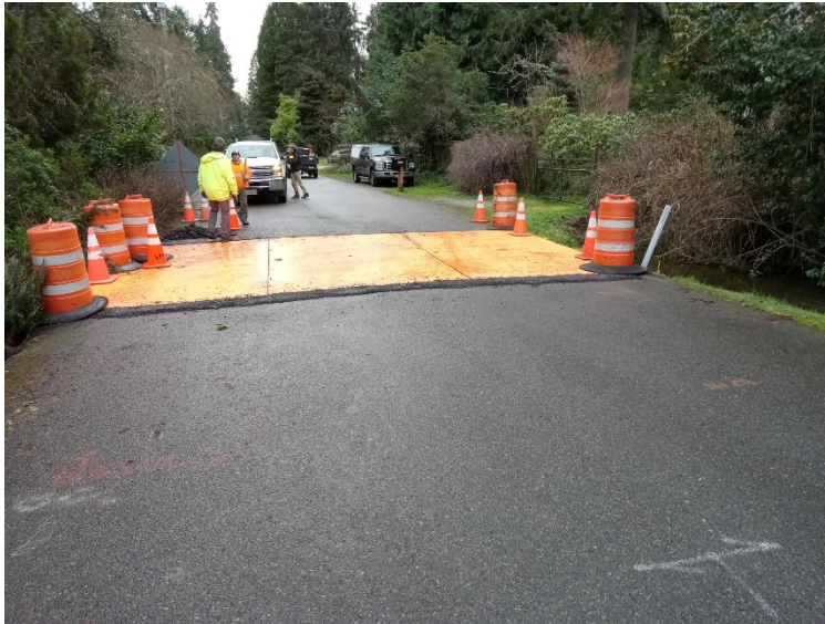
Photo: PW crew members and vendor staff complete installation of steel roadway plates
