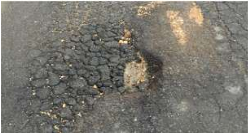
Pavement Condition 0 – 10 (Failed)
