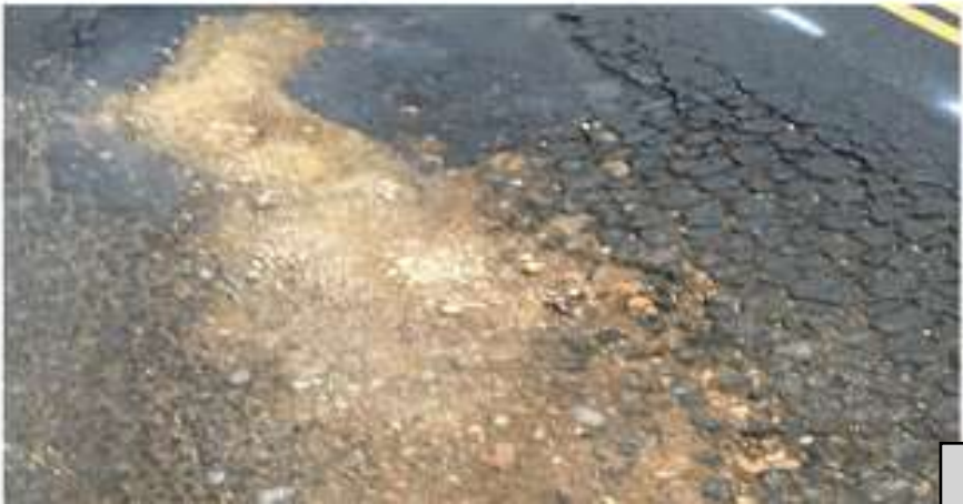
Pavement Condition 0 – 10 (Failed)
