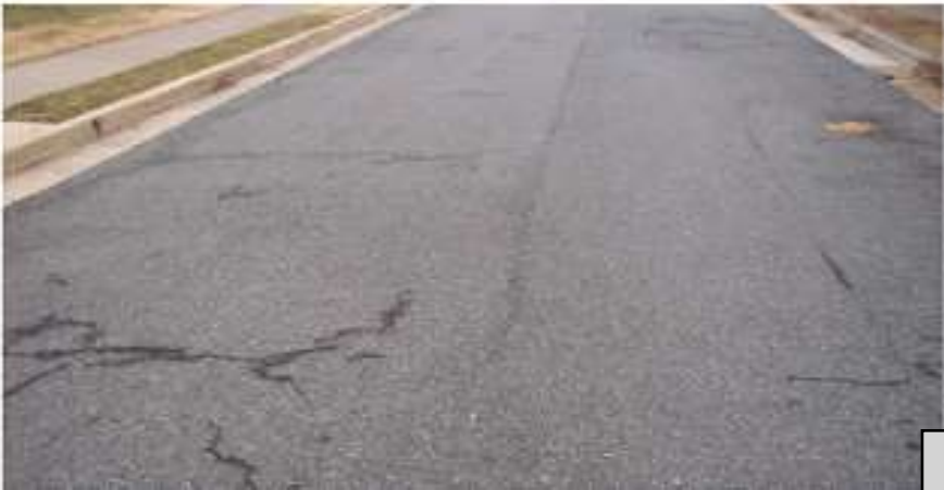
Pavement Condition 71 – 85 (Very Good)
