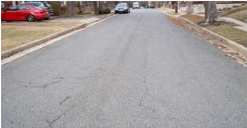
Pavement Condition 71 – 85 (Very Good)
