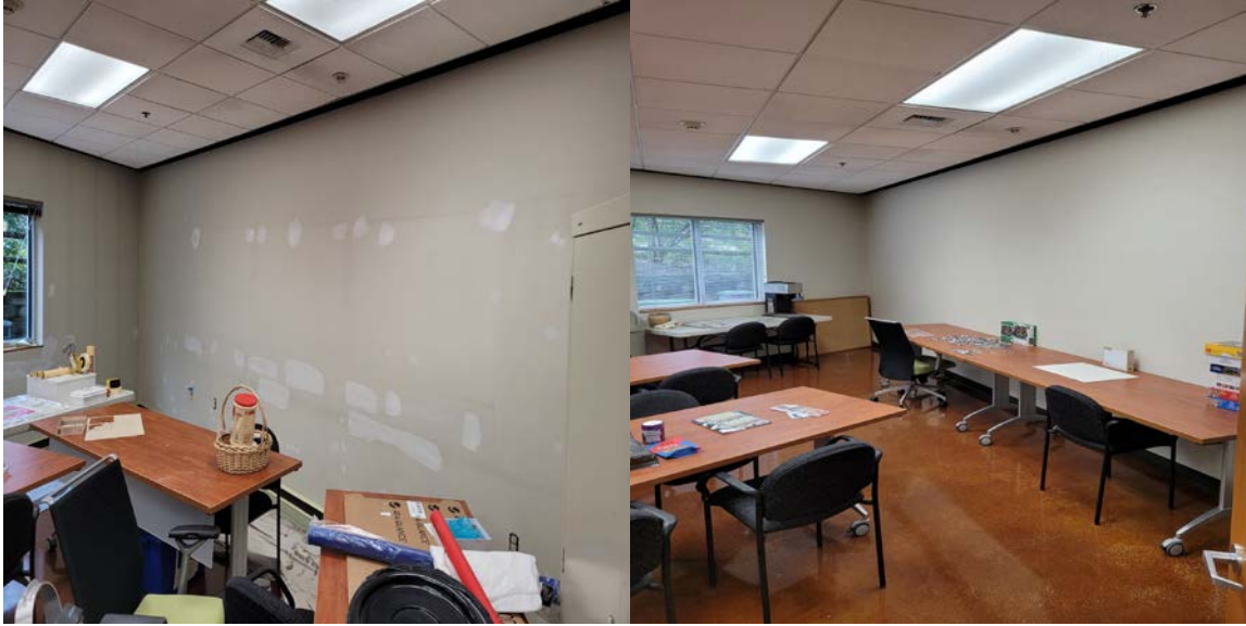
Breakroom during patching work.
